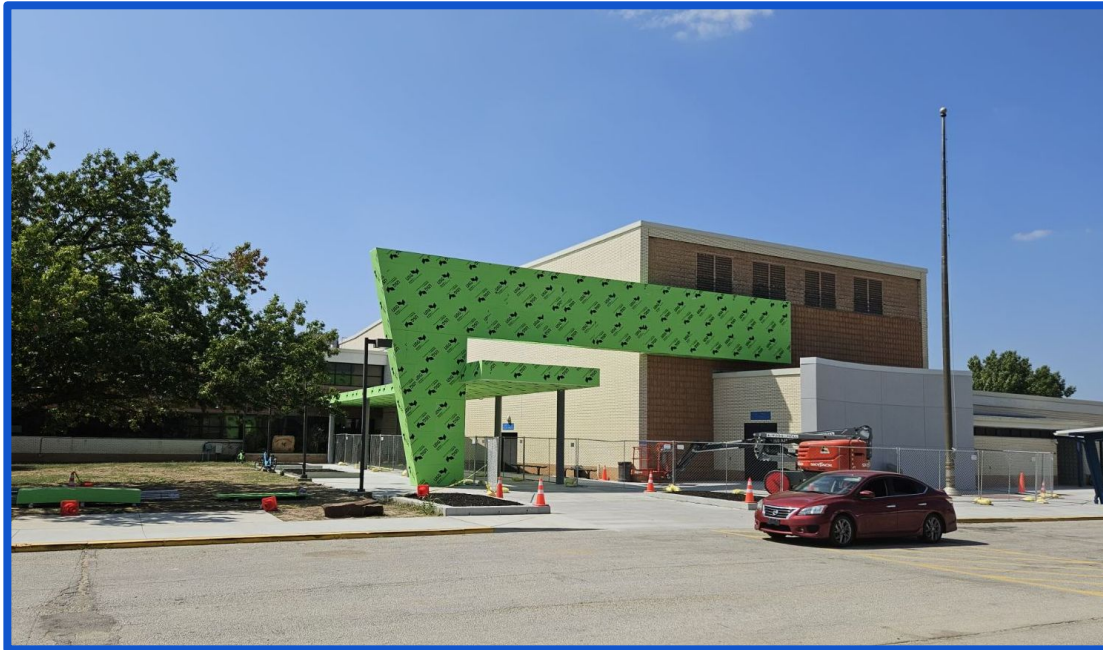
Memorial Senior High Entry ( under construction )
