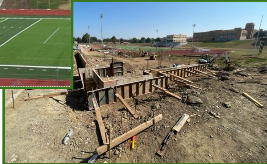
Concession stand and restrooms in progress.
