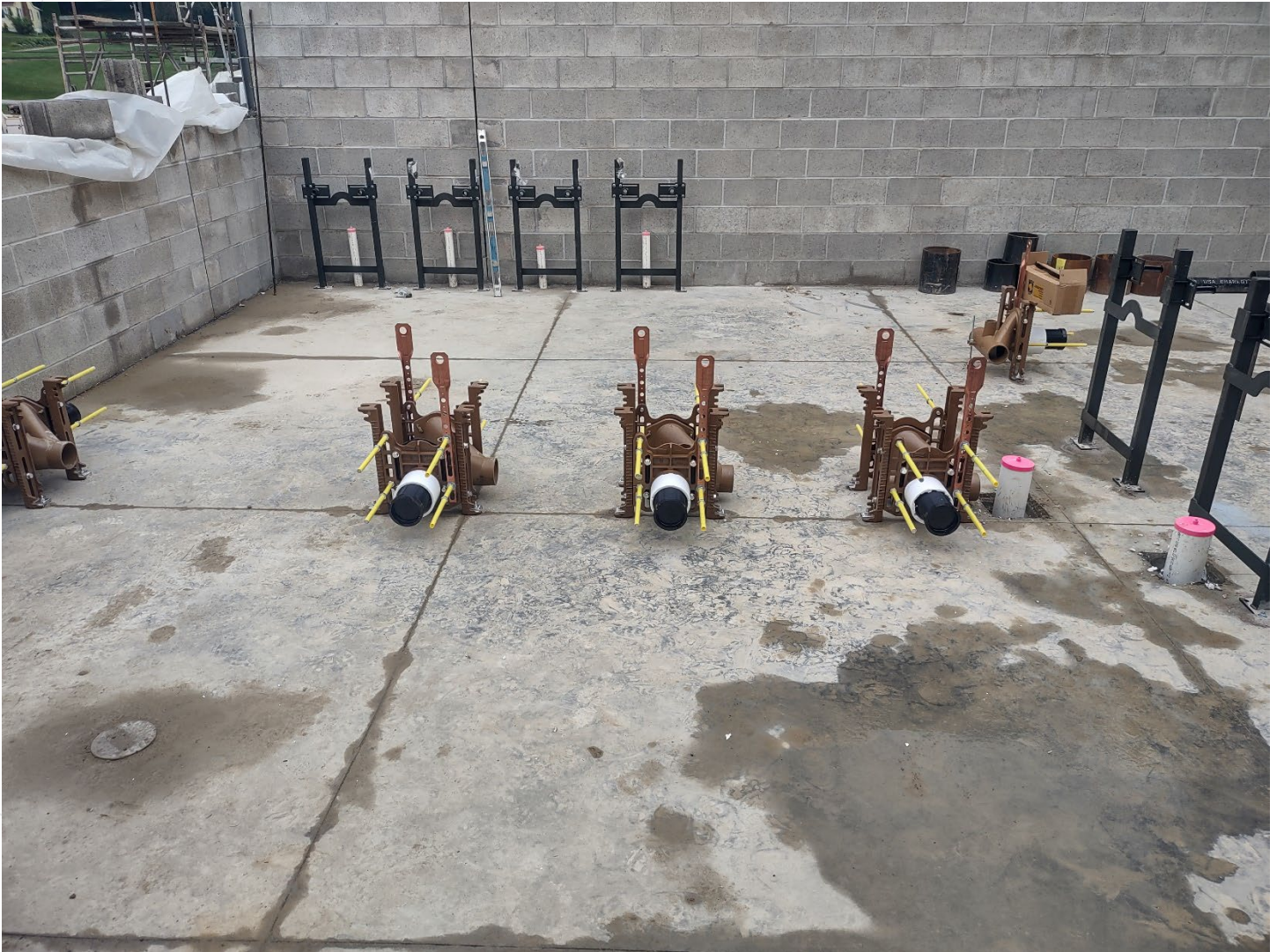
Rough-Ins for restrooms in new Classroom addition
