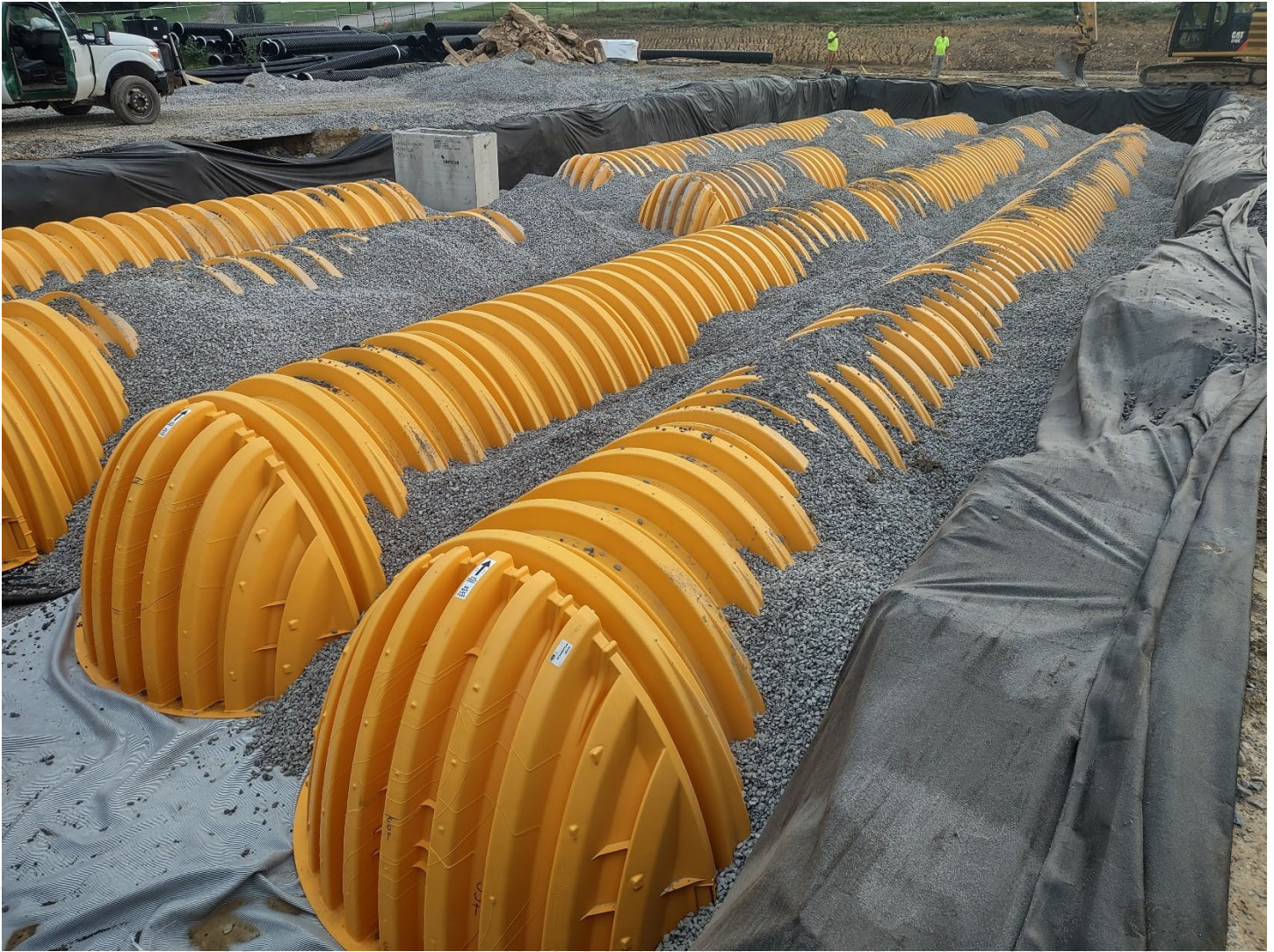
Stormwater Detention Structure along Kittaning Street
