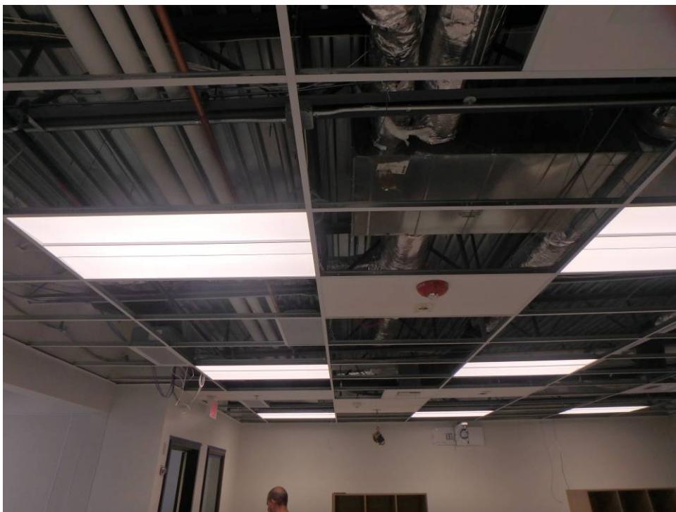
Ceiling area of the classroom
