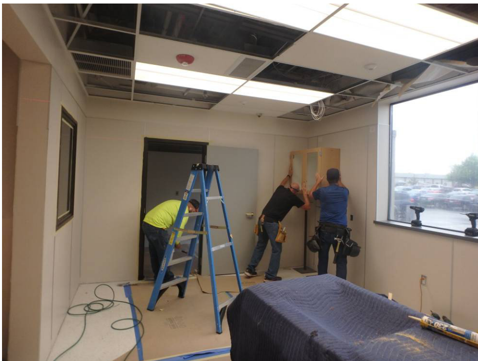
Installing casework in the southwest corner of the south exam room
