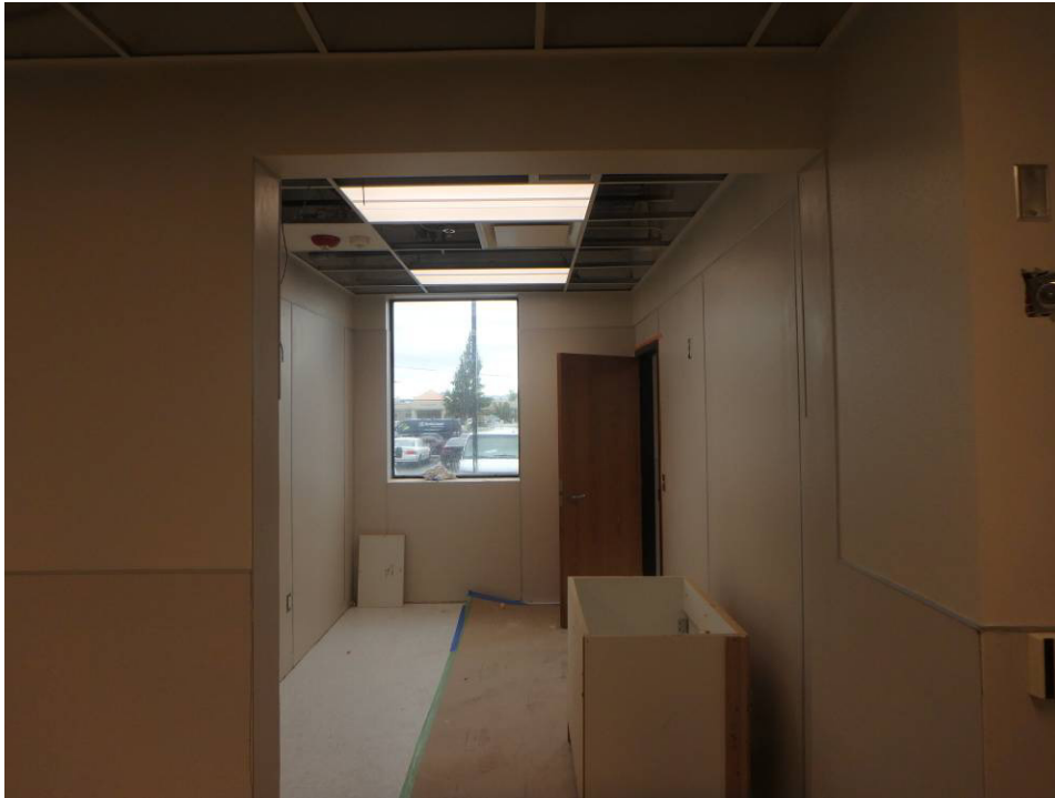
Alt. 1 main room towards north exam room
