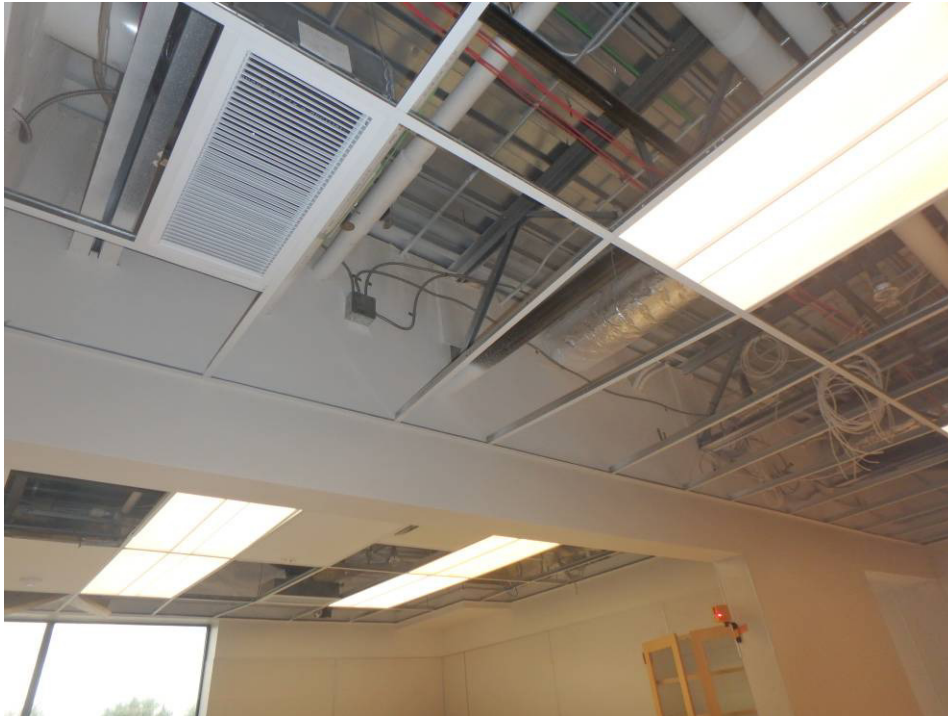
Looking west into the south exam, north end ceiling area
