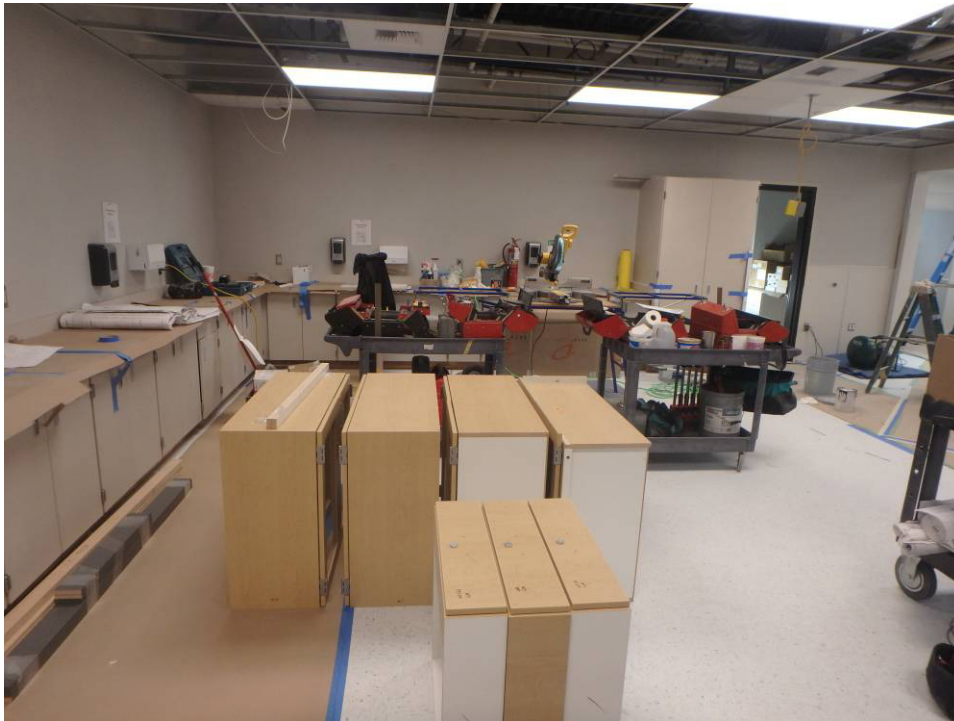
Alt. 1 main room looking south and staged casework
