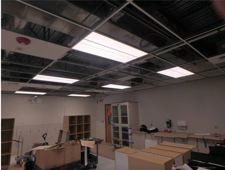
Looking northeast Ceiling area of the classroom
