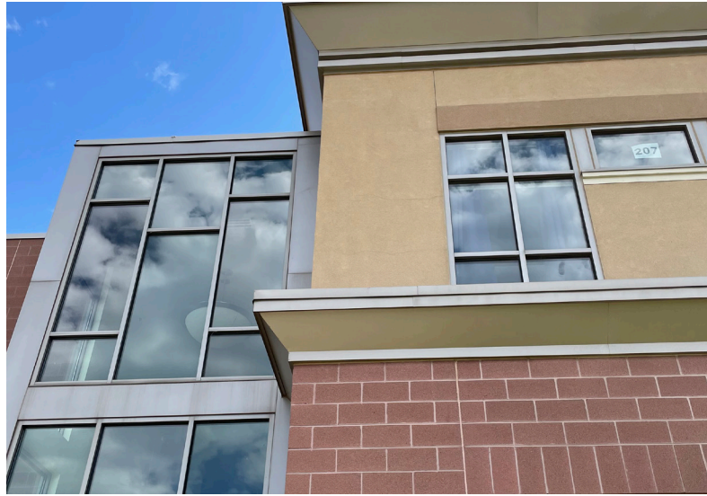
Existing exterior building
