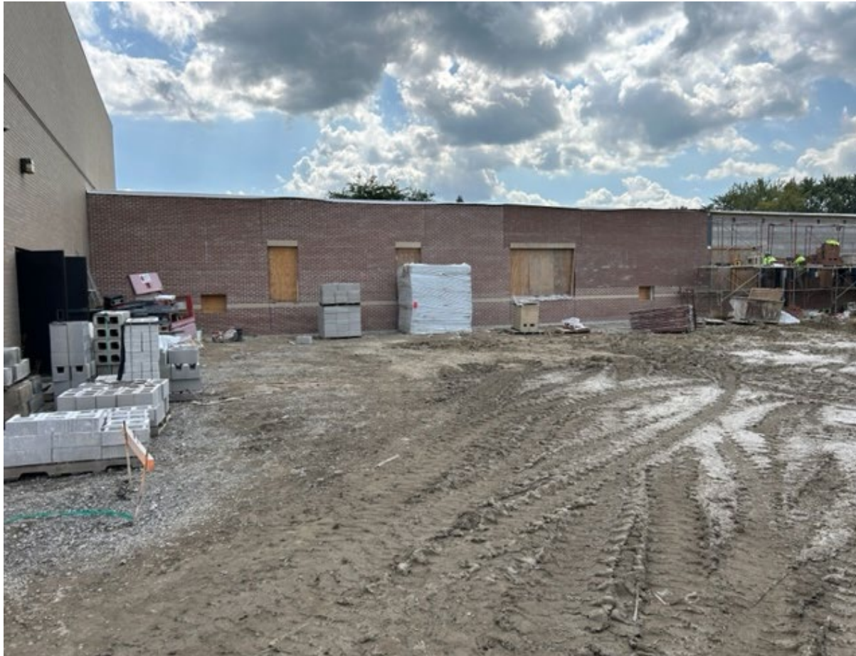
New Media Center Addition
