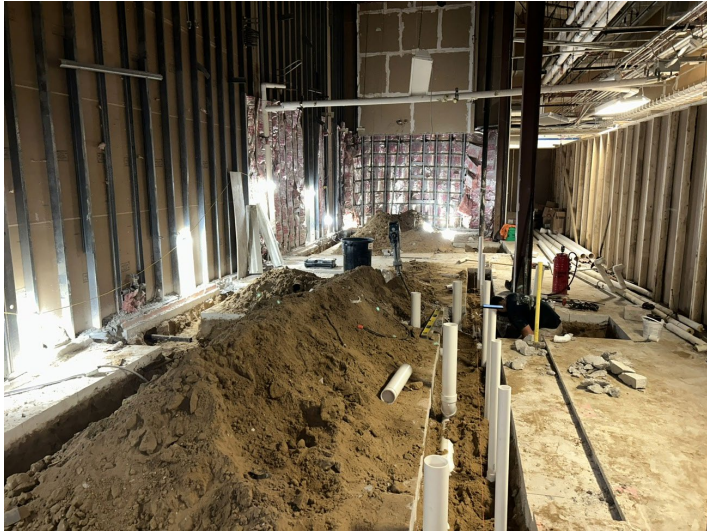
Underground Plumbing for Large Student Restrooms
