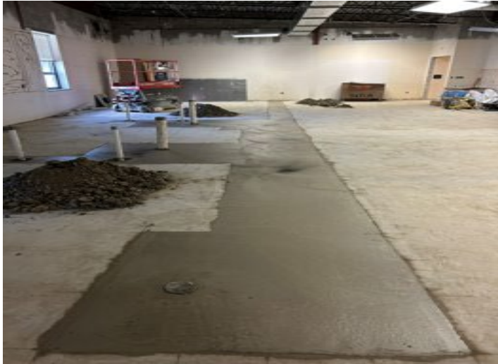
Floor Patching at Pre-K Renovation
