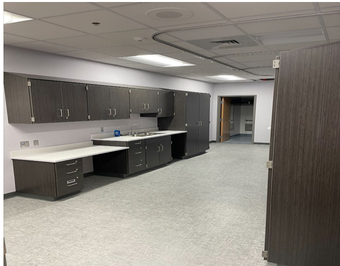
New Clinic Casework
