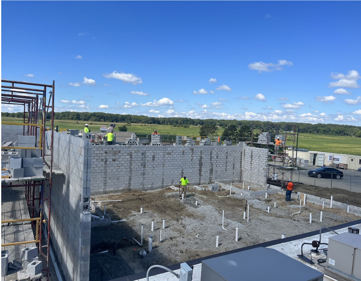
Kitchen Addition Progress
