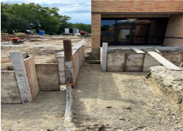
Classroom Addition Concrete Footing
