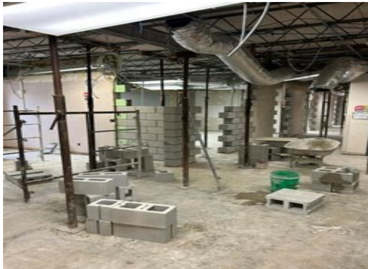
Main Entrance Renovation
