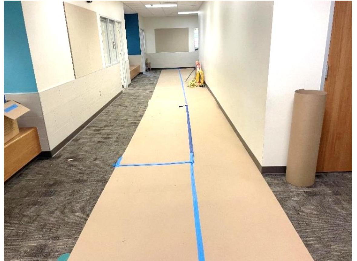
Floor protection for interior renovation
