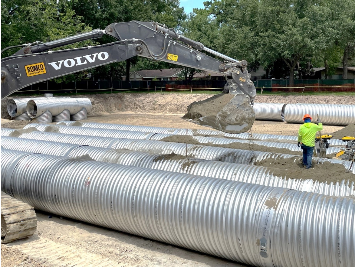
Backfilling over underground detention pipe
