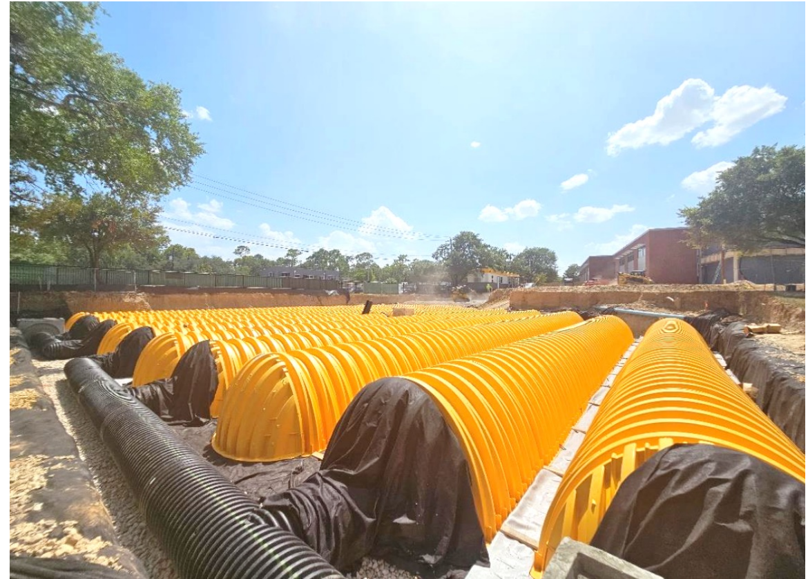
Underground stormwater detention chamber installation
