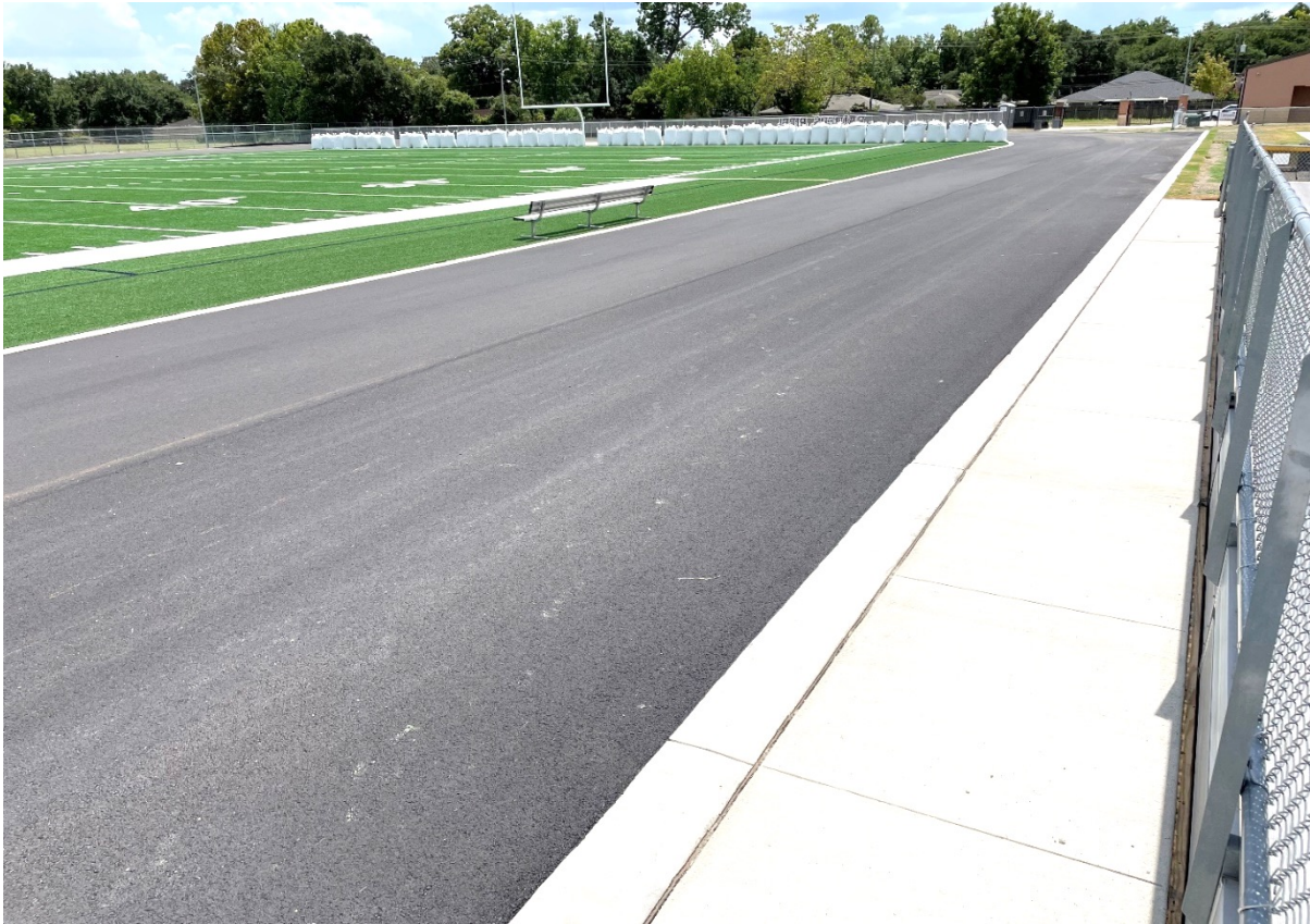
Track asphalt surface in place. Synthetic surface to be applied after football season
