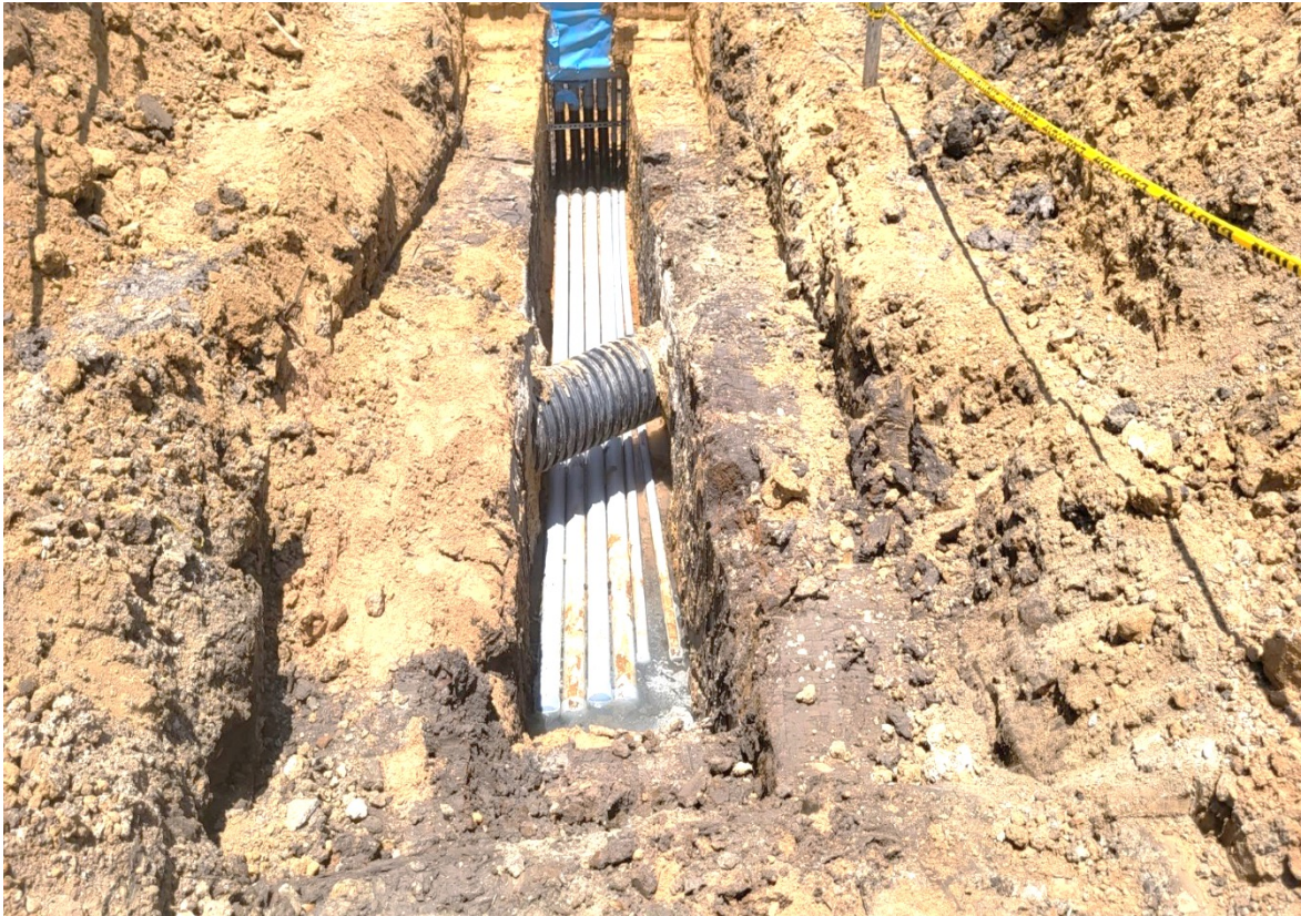
Telecommunication ductbank installation
