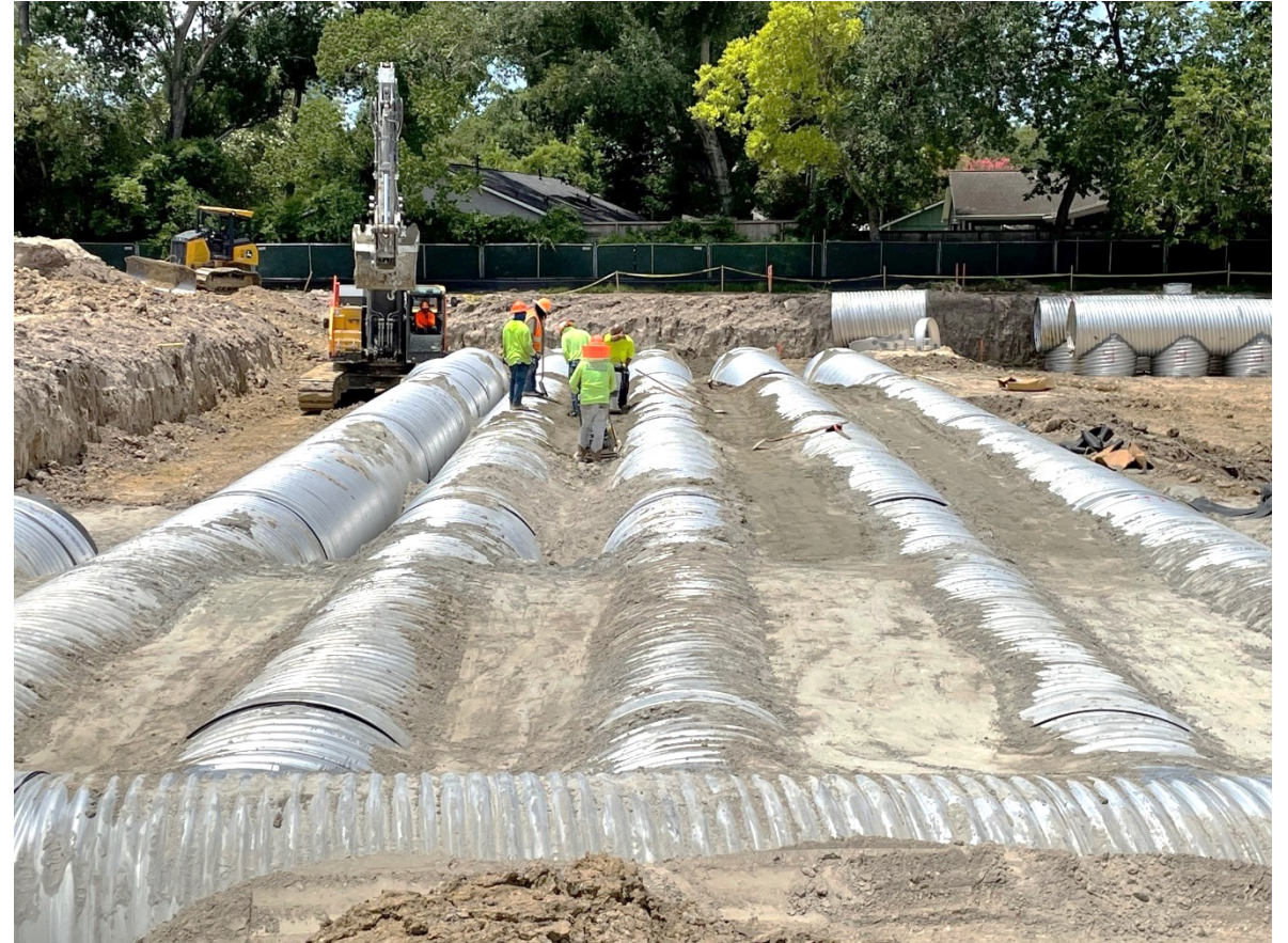
Compacted underground detention pipe
