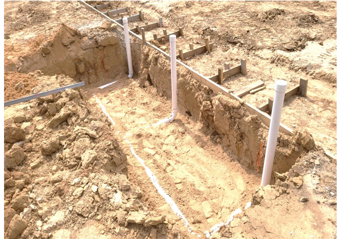
Underground plumbing installation
