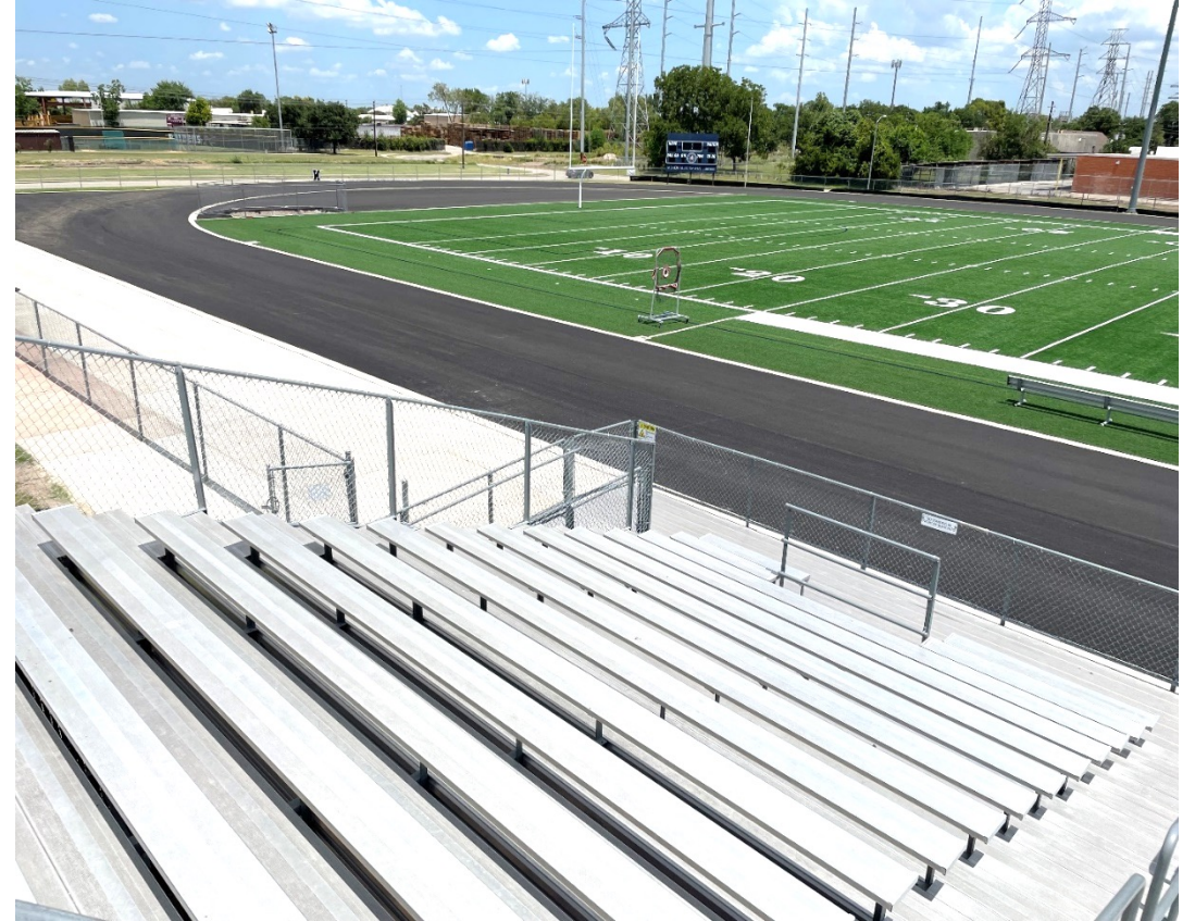
Eight lane asphalt track resized and ready for synthetic surfacing.
