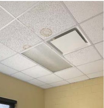
Leak in classroom ceiling
