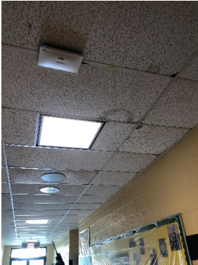
Water damage on ceiling
