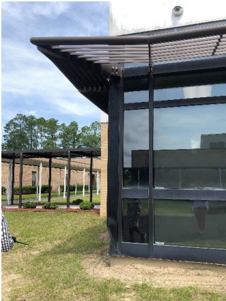
Curtain wall sunshade & downspout - corner trim dent is in need of repair
