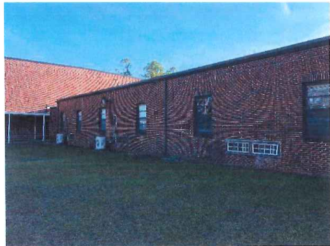
Exterior brick & thru wall mechanical units
