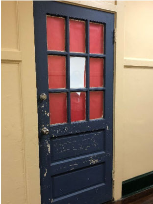
Typ. classroom door of main building – non-ADA compliant
