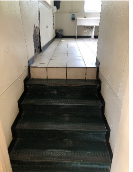
Stairs into boys group restroom in gym building – non-ADA compliant
