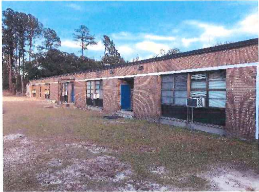
Window mechanical units at classroom wing
