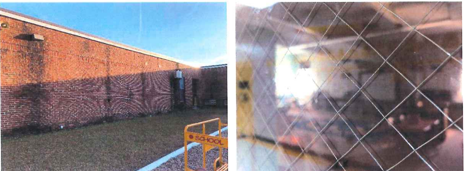
Exterior brick Wire glass (safety issue)
