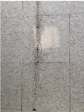
Water damage to floor in hall and control joint in flooring
