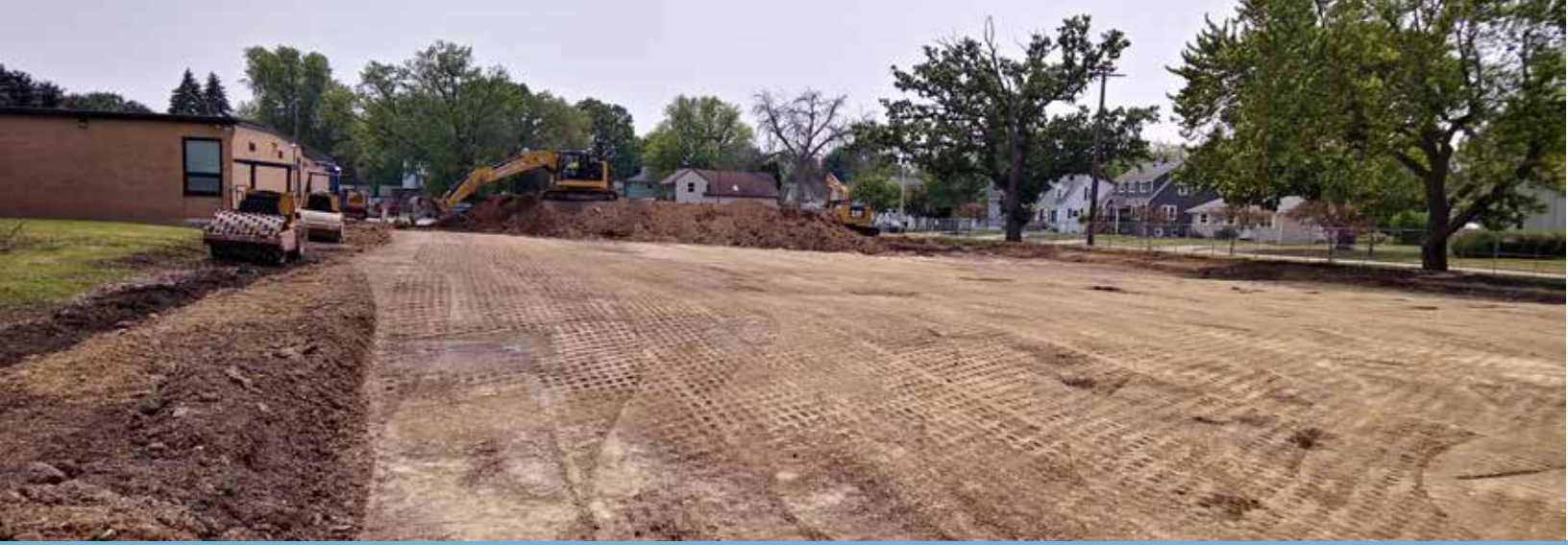
MENOMINEE ELEMENTARY SCHOOL SITE WORK UNDERWAY
