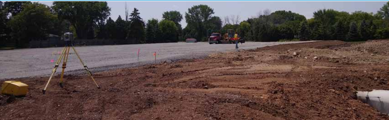
NEW OAKWOOD ELEMENTARY SCHOOL PARKING LOT
