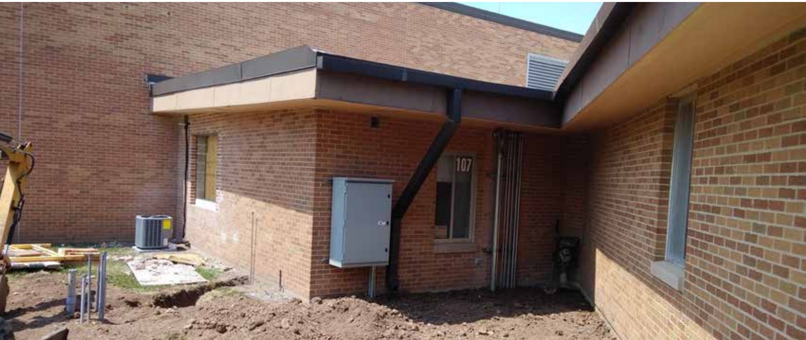
OAKWOOD ELEMENTARY SCHOOL NEW WINDOW AT HEALTH AND GENERATOR PREPARATION
