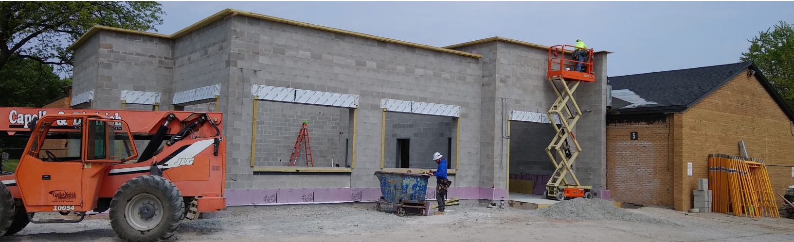
OAKWOOD ELEMENTARY SCHOOL ADDITION BEARING WALLS FINISHED
