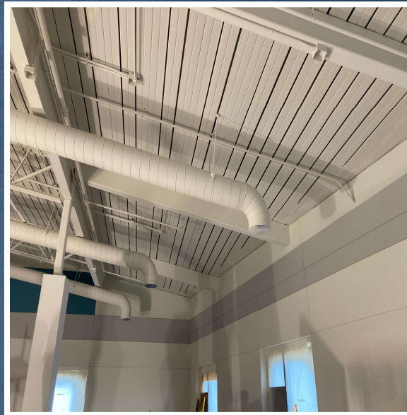
Library & Computer Room Painted
