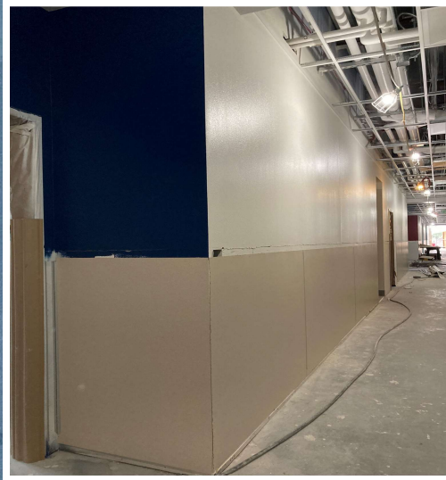
Corridor FRP in Progress
