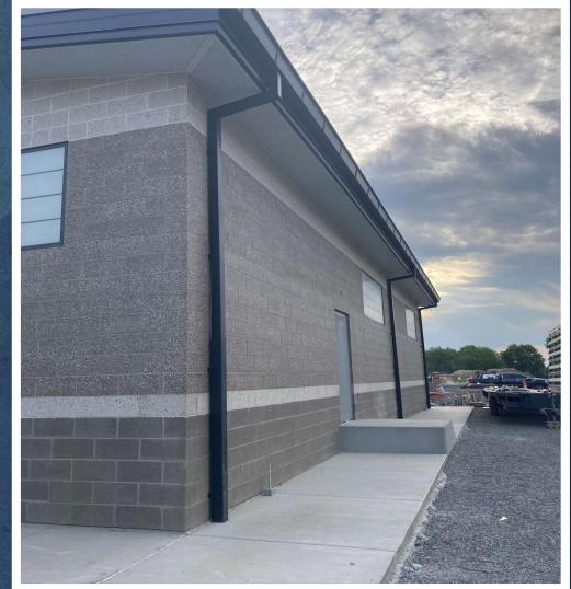
Downspouts Installed
