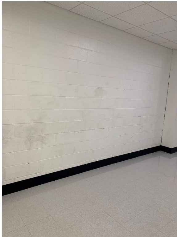
Ground level hallway – Staining on CMU walls shown. No obvious/suspect mold/mildew growth noted at the time of the assessment.
