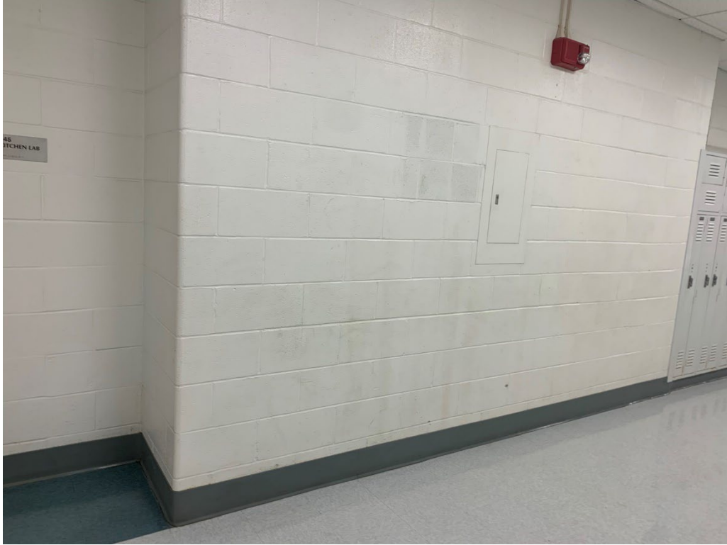
Ground level hallway – Staining on CMU walls shown. No obvious/suspect mold/mildew growth noted at the time of the assessment.
