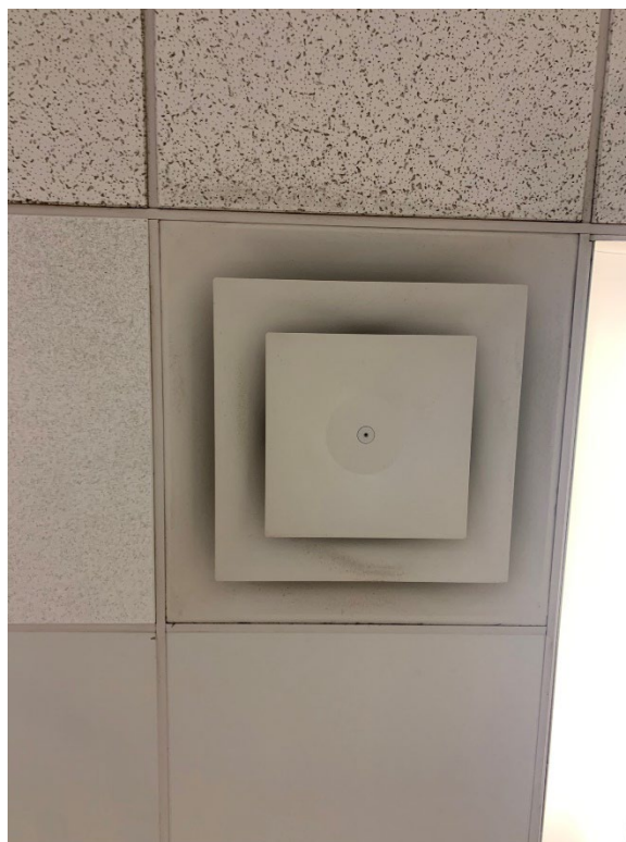
Room 149 classroom - HVAC diffuser and adjacent suspended ceiling tile with built-up dust and/or possible mold.
