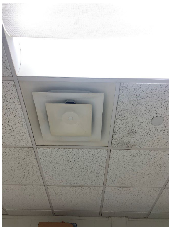
Room 153 Physics - HVAC diffuser and adjacent suspended ceiling tile with built-up dust and/or possible mold. Water stained ceiling tile shown.
