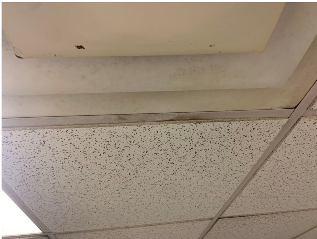
Room 151 Physics - HVAC diffuser and adjacent suspended ceiling tile with built-up dust and/or possible mold.
