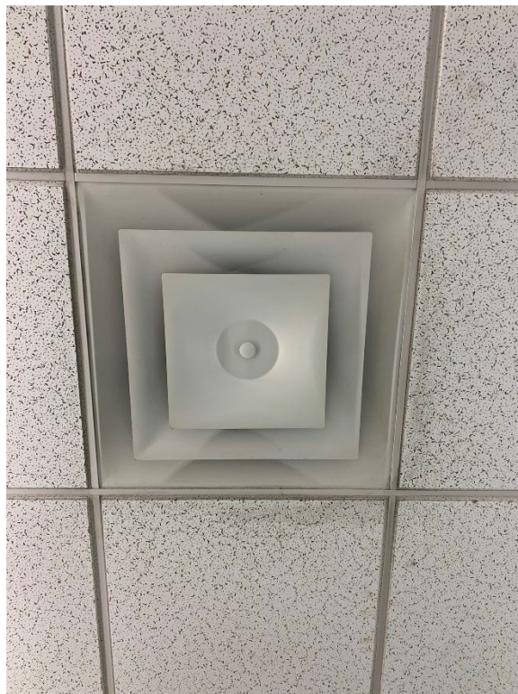
Room 150 Computer Lab - HVAC diffuser and adjacent suspended ceiling tile with built-up dust and/or possible mold.
