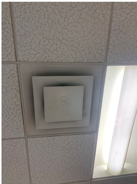
Room 148 classroom – HVAC diffuser with built-up dust and/or possible mold.
