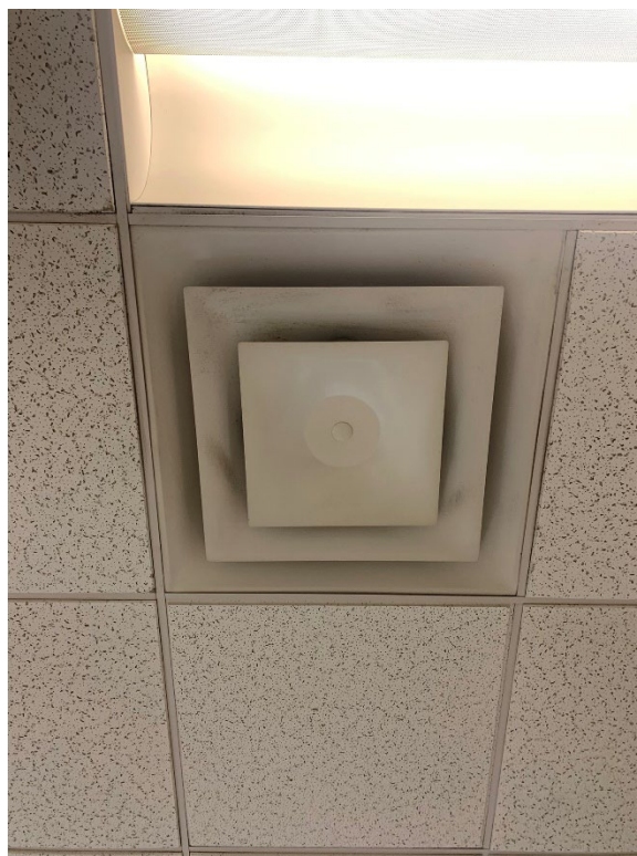
Room 147 classroom - HVAC diffuser with built-up dust and/or possible mold.
