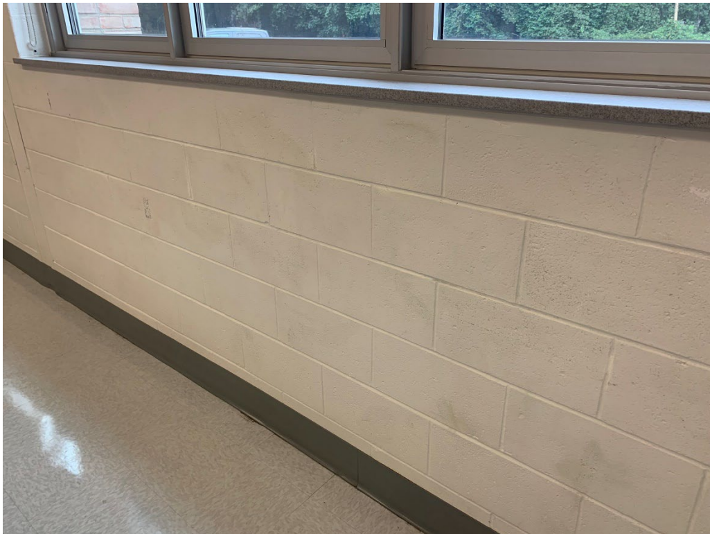
Room 148 classroom - Staining on CMU walls shown. No obvious/suspect mold/mildew growth noted at the time of the assessment.
