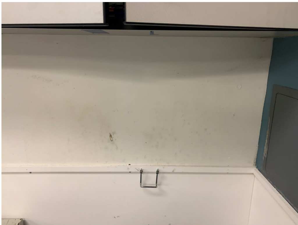
Room 153 Physics – Staining on gypsum wall in southeast corner of room.
