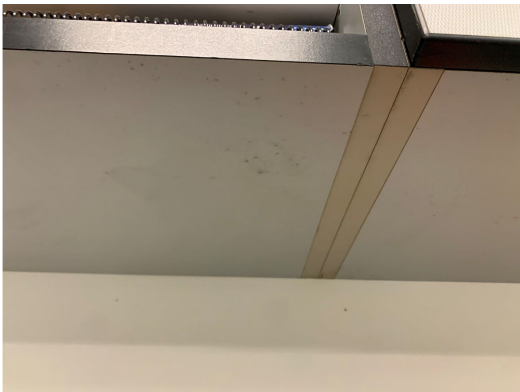
Room 151 Physics – Suspect mold below upper cabinets.
