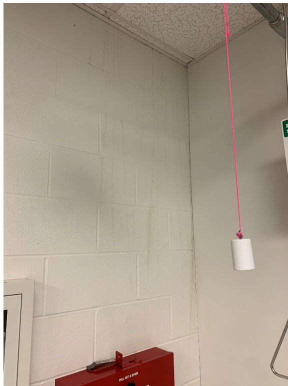
Room 153 Physics – Water staining (drips) on CMU wall.
