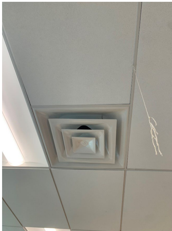
Room 181 Science Room – Typical HVAC diffuser vent.
