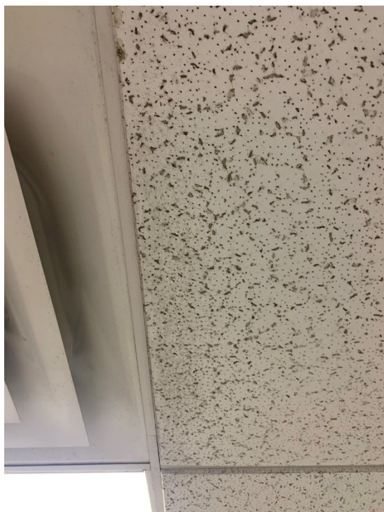
Room 148 classroom – Staining (dust build-up and/or possible mold) observed on suspended ceiling tile adjacent to HVAC diffuser (typical).
