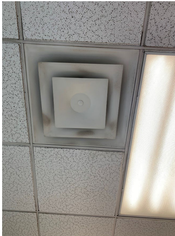
Room 145 Kitchen Lab - HVAC diffuser with built-up dust and/or possible mold.
