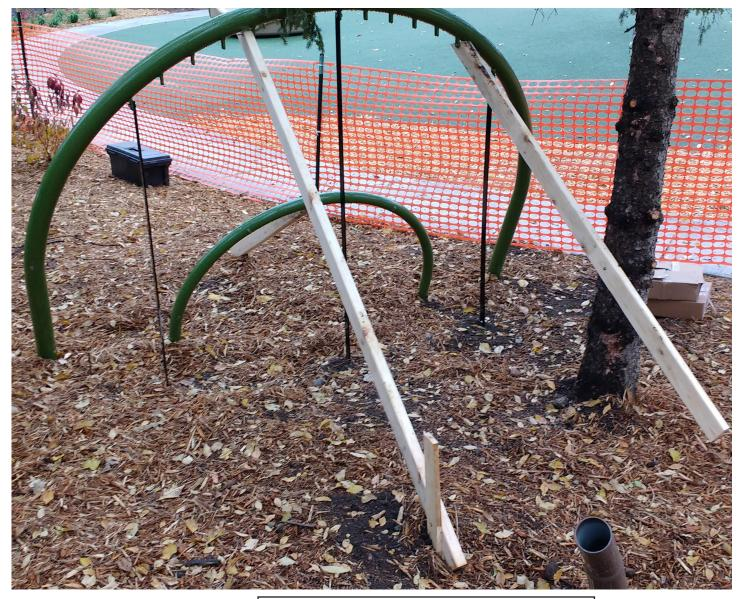
NOTE: Picture shown is an example of how to prop the frame and mallet bar in final position, using 2 x 4 boards and wooden stakes, prior to pouring concrete footings.
