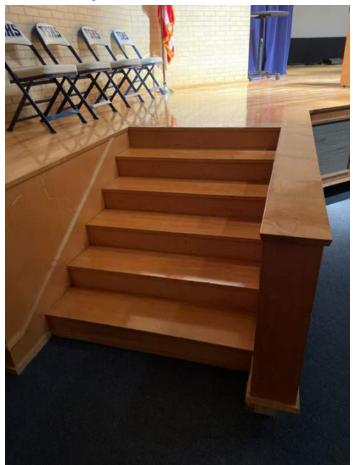
Building Codes - 7. Stage, stage storage, and changing rooms are not fire rated. Current code requires this stage to have 2 hour separation and the other spaces to have one hour separation.
