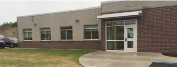
The public entrance for the new transportation center is on the west side of the building.
