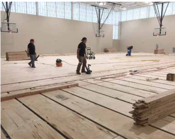
Construction at Phoenix High School includes a new gym, a courtyard off of the cafeteria, additional classrooms, and a support services center.
