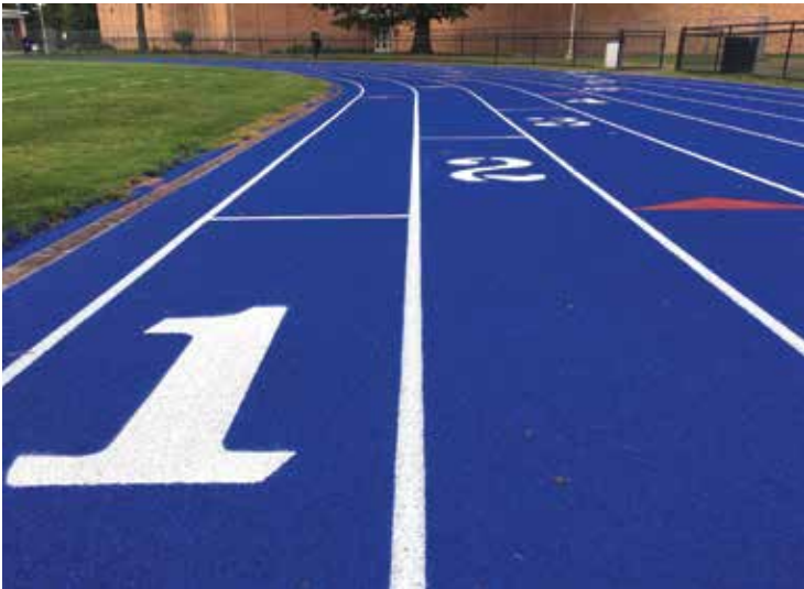
Construction at Loy Norrix included the installation of a new track, new tennis courts, and a new softball diamond.
