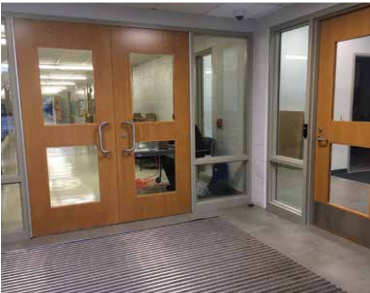
The district construction this summer included five new secure vestibules at Northeastern, Winchell, Greenwood, Arcadia, and this one at King-Westwood elementary.
