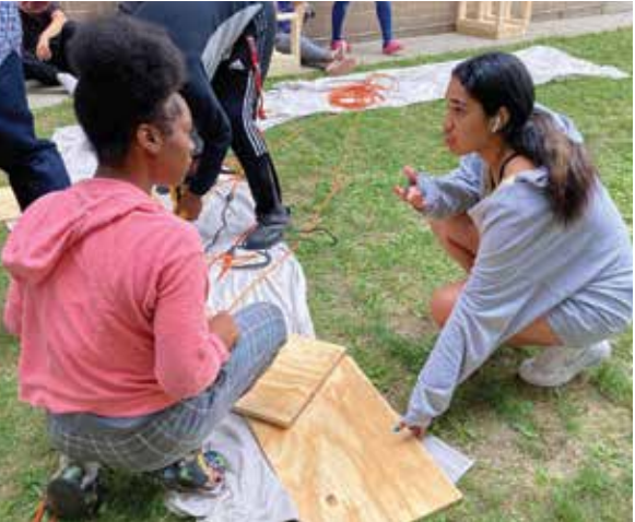
Armani Pompey talks to Shakira Bailey about the next steps to take on building their doghouse.
