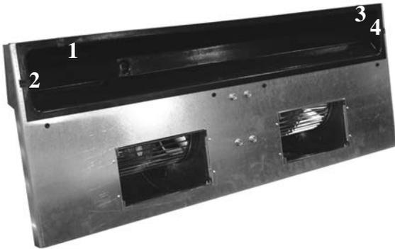
**Access to Fanboard & Motor.** The unit ventilator fan board can be removed for service to the blower motor and fan wheels. The fan board must also be removed for easier access to the unit coils for cleaning and maintenance. Utilize the following steps for proper removal of the fanboard.
