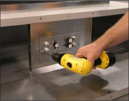
D. Pull the power wires from inside the heat pump, through the electrical bushing. Connect the wires as shown in the electrical diagram that is on the heat pump.
