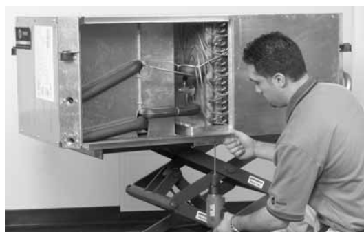
Figure 21. Install top/bottom filter rack
