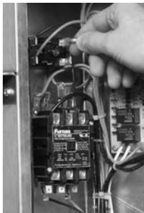
Figure 63. Connecting speed-tap wire
