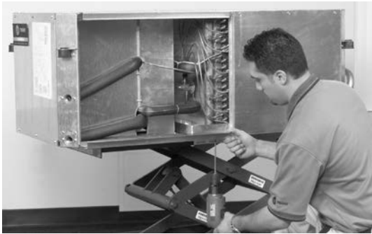
Figure 51. Install top/bottom filter rack
