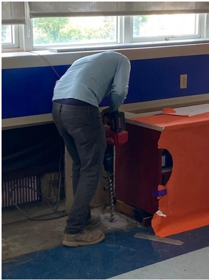
Image Description: (left) the mechanical contractor is drilling holes in the floor slab for new piping, (right) remnants of a removed unit ventilator, awaiting new equipment.
