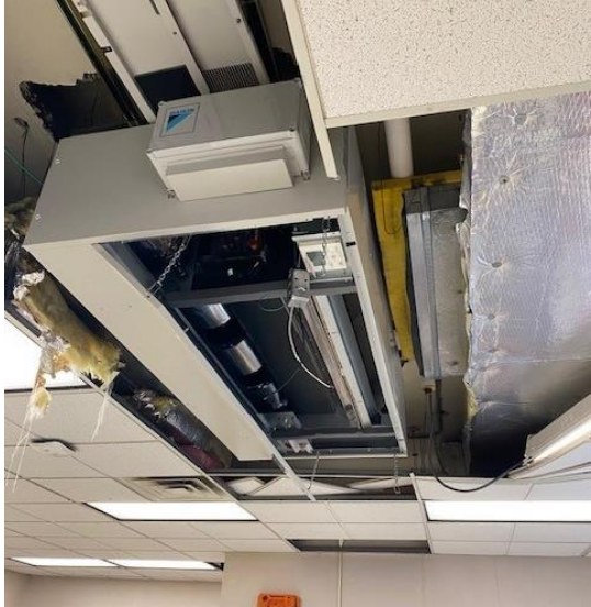
Image Description: (left) a ceiling hung unit ventilator being removed in 'G'-Wing, (right) a ceiling mounted new unit ventilator being installed in 'G'-Wing.
