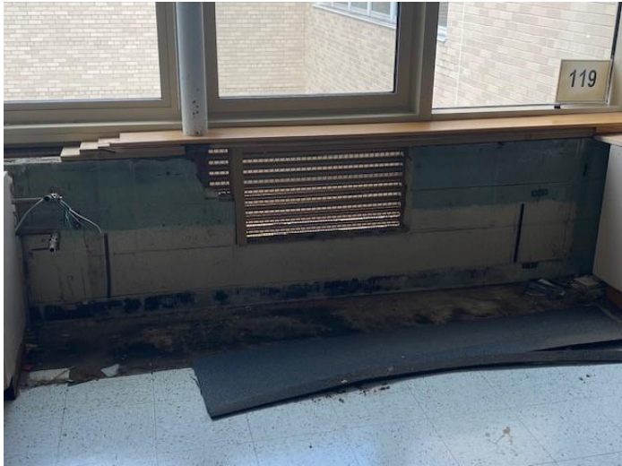
Image Description: (left) the mechanical contractor is drilling holes in the floor slab for new piping, (right) remnants of a removed unit ventilator, awaiting new equipment.
