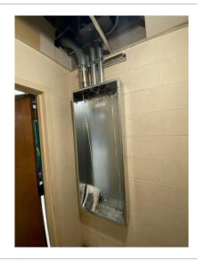
**Image Description:** (left) remnants of unit ventilator that has been removed, awaiting a new air louver to be installed in it's façade and (right) a new electrical panel housing, awaiting internal components.
