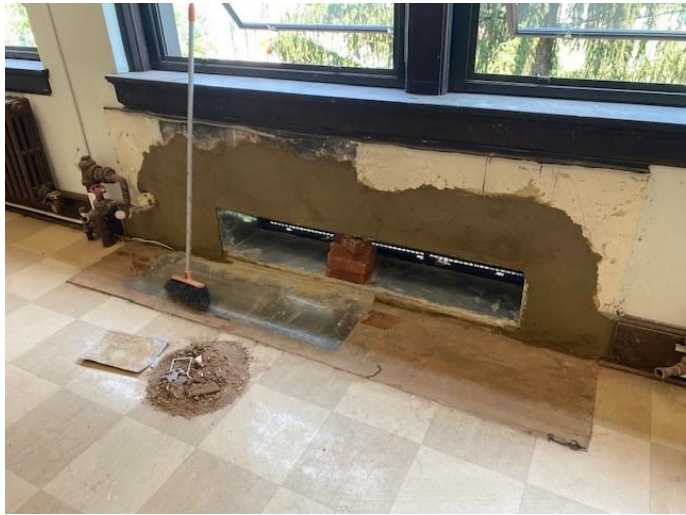
Image Description: (left) the remnants of what is left after a unit ventilator is removed (i.e.: louver/ wall/ flooring), (right) the a new unit ventilator installed, awaiting final terminations.
