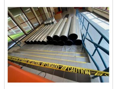
**Image Description:** (left) a new standing "TempSpec" Unit Ventilator, recently received and being staged for installation, (right) with new round ductwork- which will be installed in a number of classrooms.
