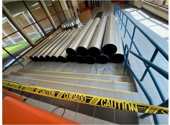
Image Description: (left) a new standing “TempSpec” Unit Ventilator, recently received and being staged for installation, (right) with new round ductwork- which will be installed in a number of classrooms.
