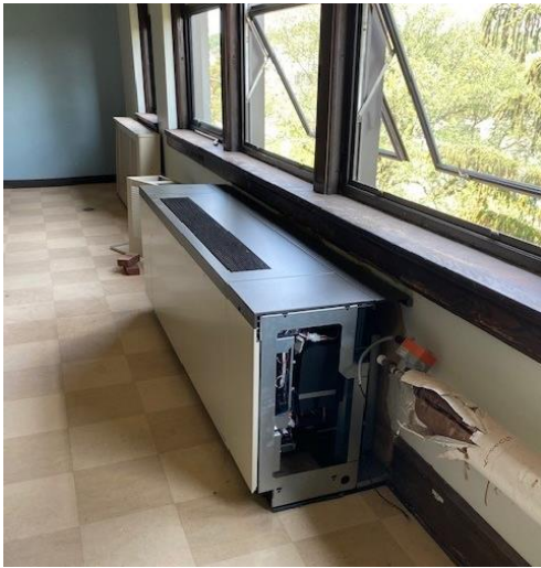
Image Description: (left) the remnants of what is left after a unit ventilator is removed (i.e.: louver/ wall/ flooring), (right) the a new unit ventilator installed, awaiting final terminations.
