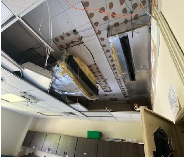
Image Description: (left) a ceiling hung unit ventilator being removed in 'G'-Wing, (right) a ceiling mounted new unit ventilator being installed in 'G'-Wing.
