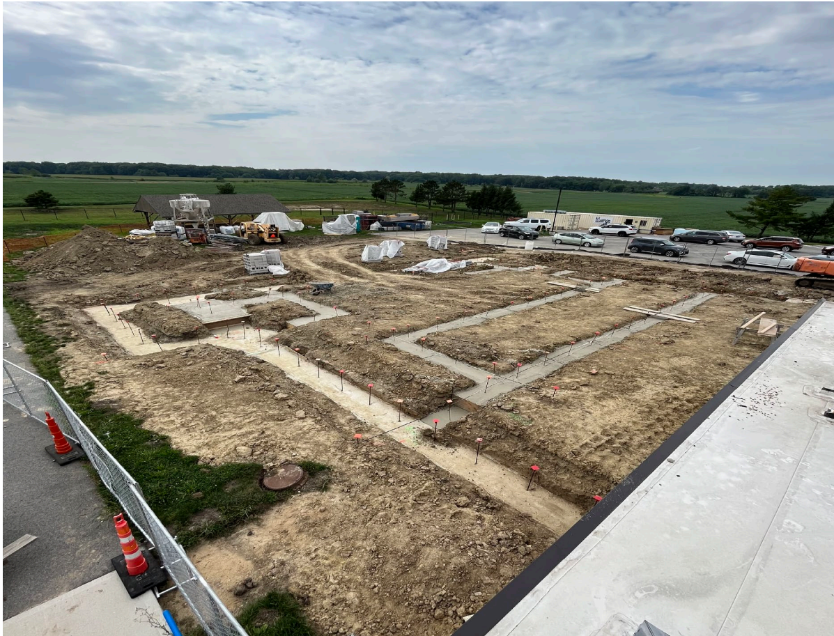
Concrete Footings for Kitchen Addition
