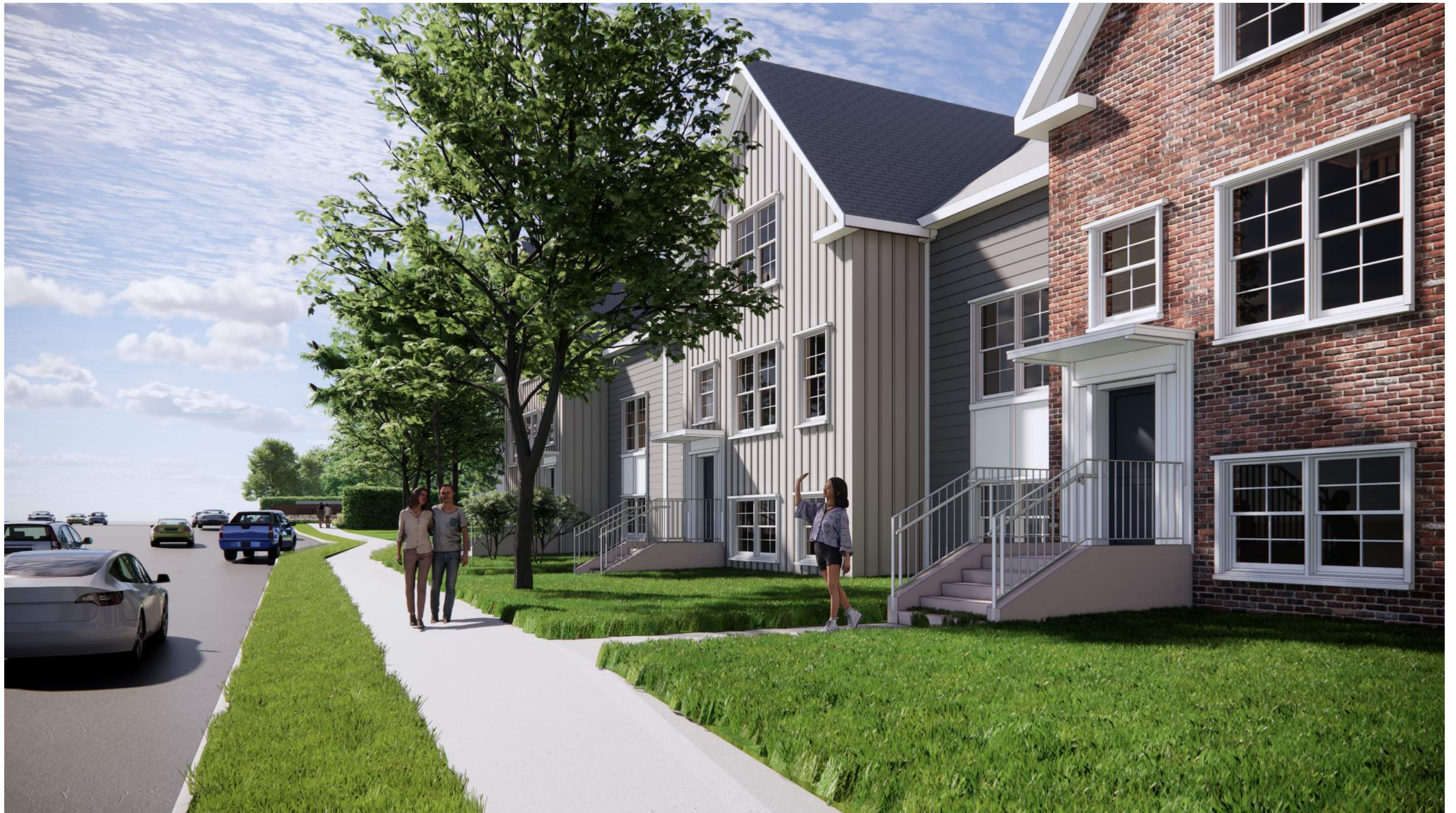
View of Asylum Avenue Townhouses Looking West (Buildings 7)
