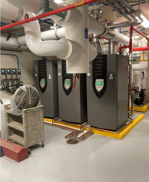
Madison Elementary - Replaced boilers with new high efficiency boilers. (photo to the left)
