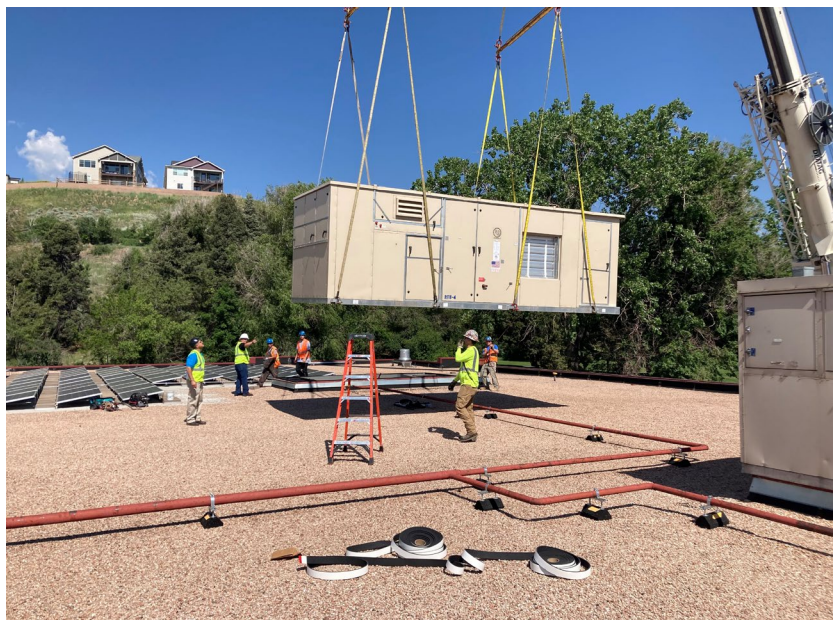
Bristol Elementary - Replaced all roof top units (RTU) that have a higher EER, thus saving the district energy dollars, along with new high efficiency motors on all return fans. (photo to the right)
