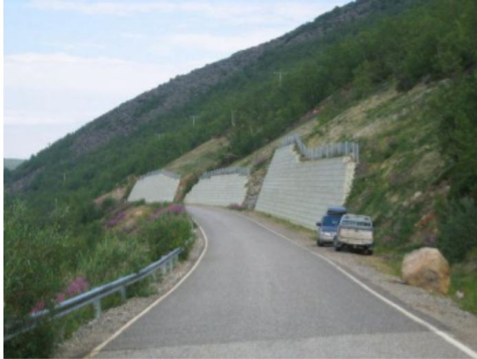
A rock wall stabilizes a slope that has been cut away to make a road. Retaining walls in Finland Utsjoki by Timo Saarenketo, https://flic.kr/p/edQe41 , CC-BY
