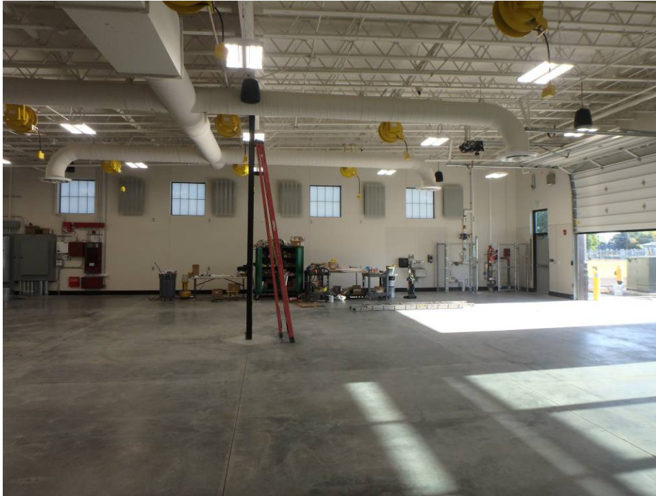
Shop – north half looking north (8/14)
