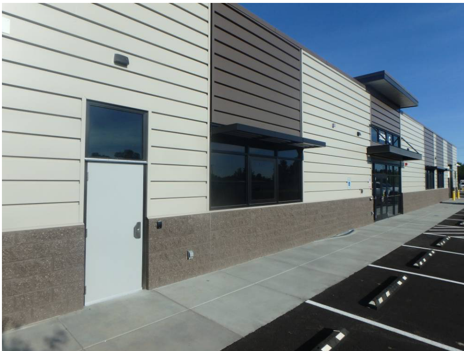
Looking north along the front sidewalk
