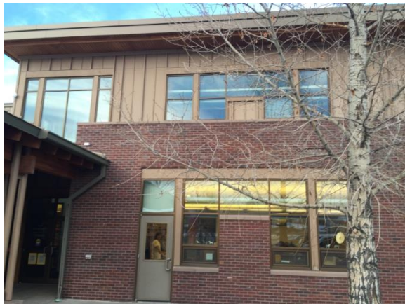
Exterior brick veneer and metal panel.
