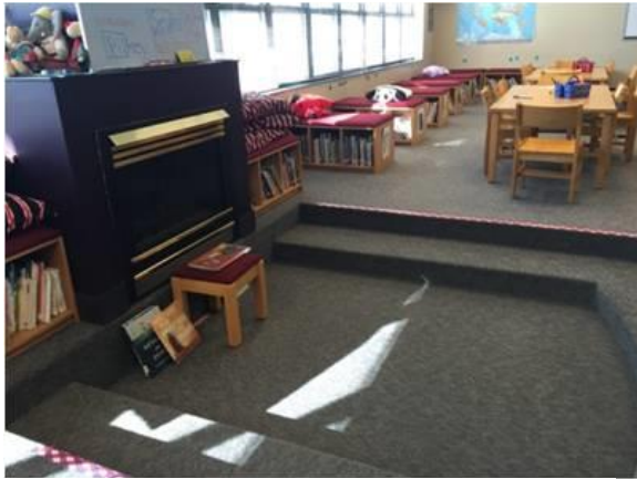
In the Media Center, the sunken story-time area creates a safety concern for tripping/falling
