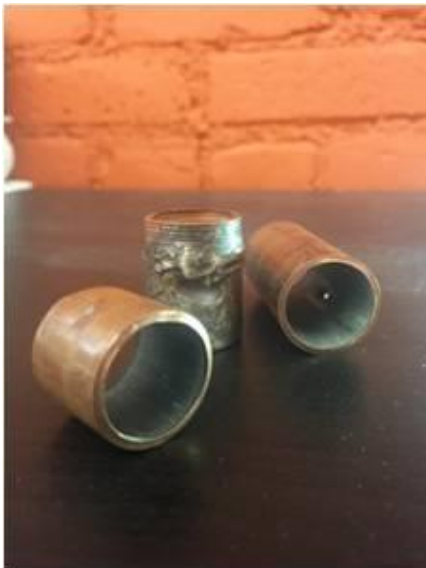
Domestic hot water piping has had pinhole leaks which required sections of the pipes to be replaced. The underlying cause of this has not been determined
