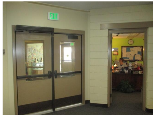
Main entrance vestibule doors and Main Office. The Office is very small and has limited visual access to the building entrance. There is not a secure vestibule to check-in visitors before they enter the school.
