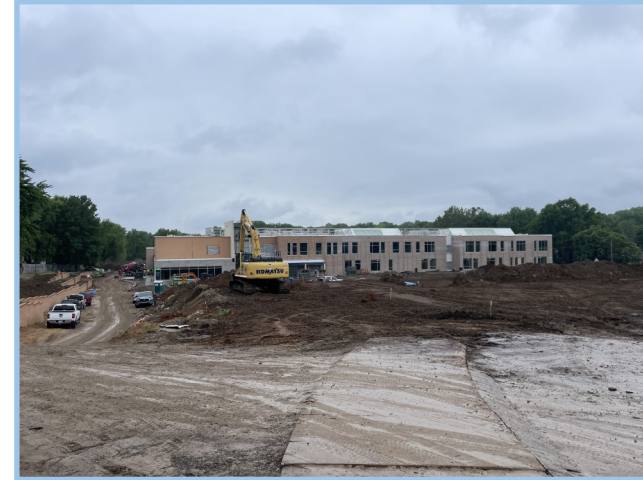
Mass Grading at North Side
