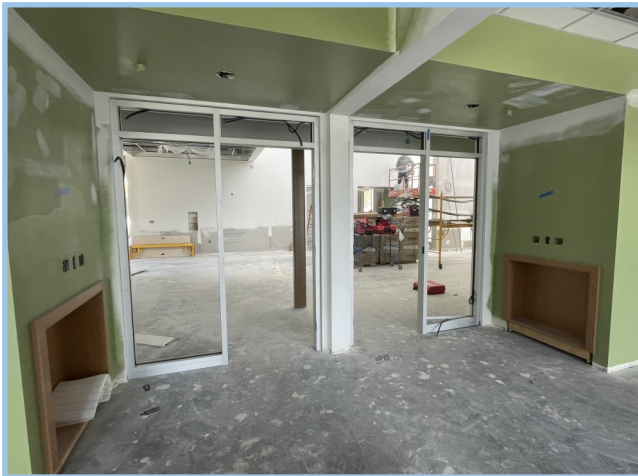
Interior Aluminum Frame Install
