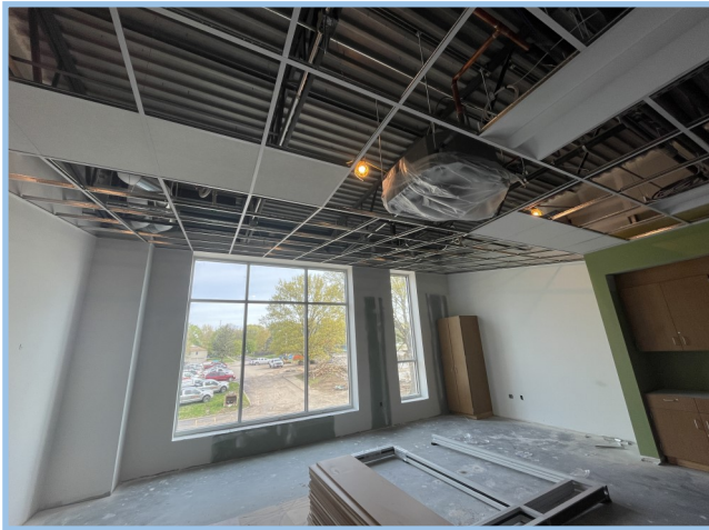
Ceiling Grid Install
