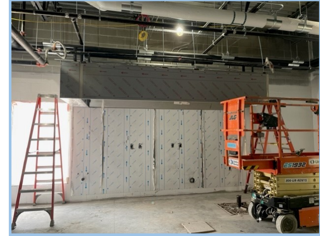
Stainless Steel Panel Install
