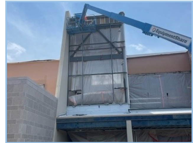
Front Entrance Curtain Wall Install
