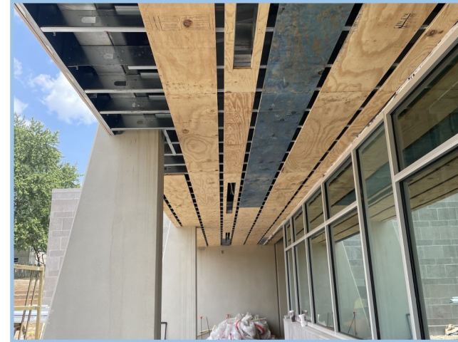
Soffit Venting at Front Entrance
