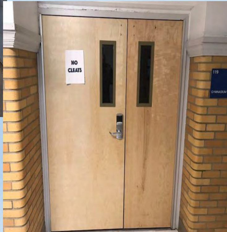
Middle School Interior Door Replacement
