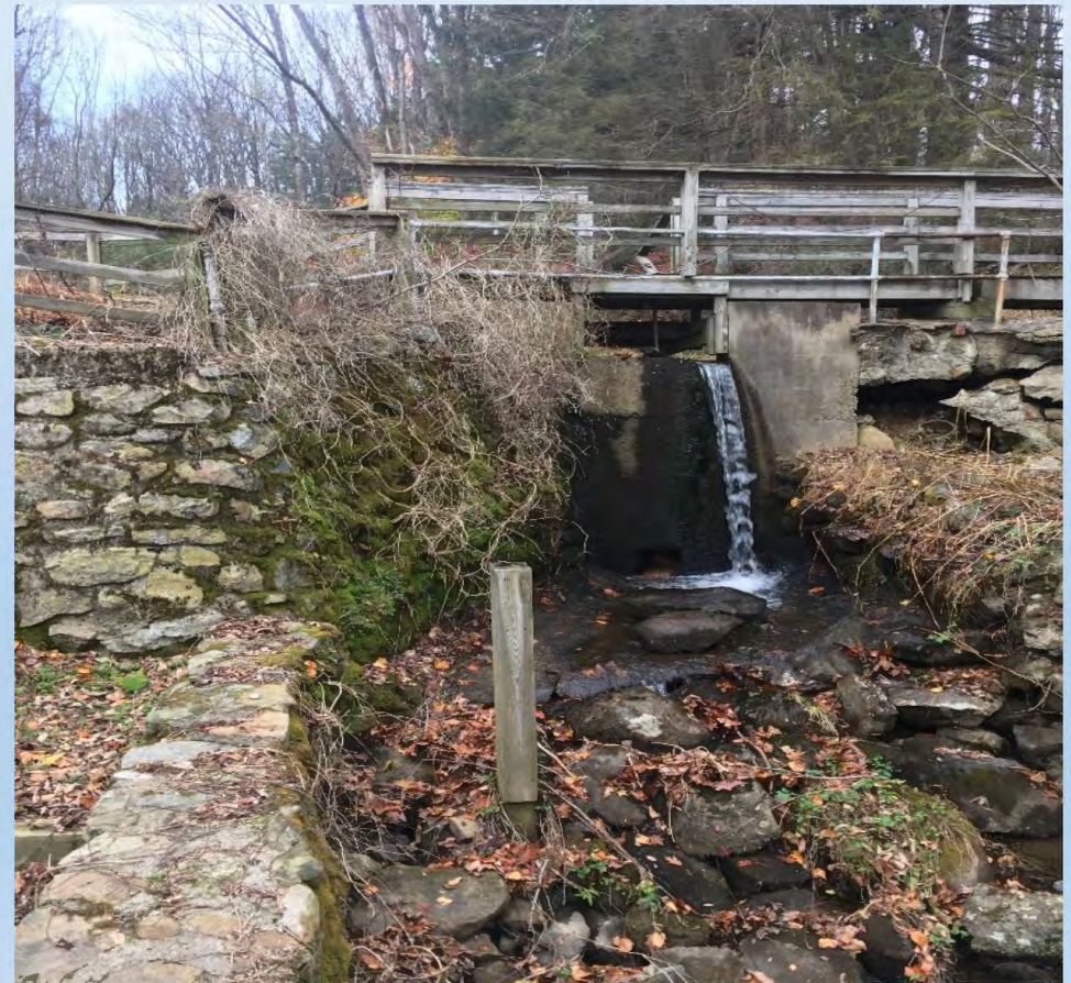
Decommission of Dam
