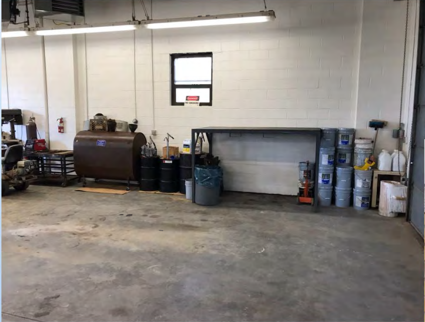
Painting of Maintenance Garage
