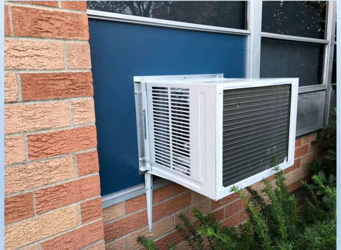
Installation of Air Conditioner Units at the High School & Middle School
