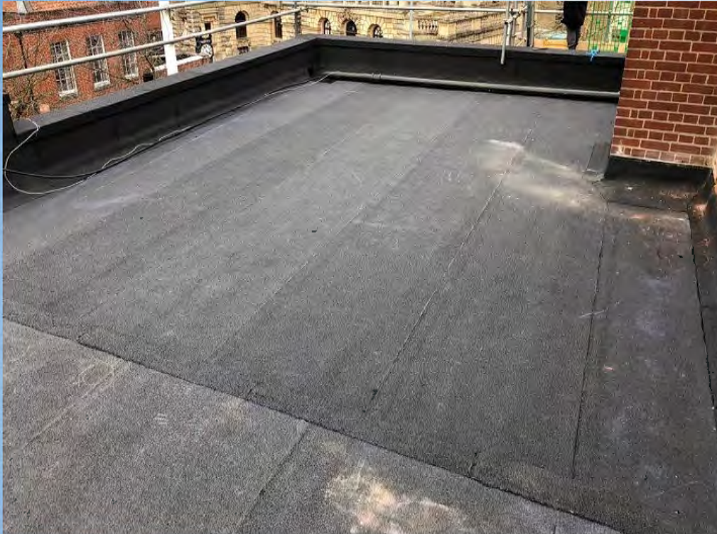
Partial Roof Replacement
