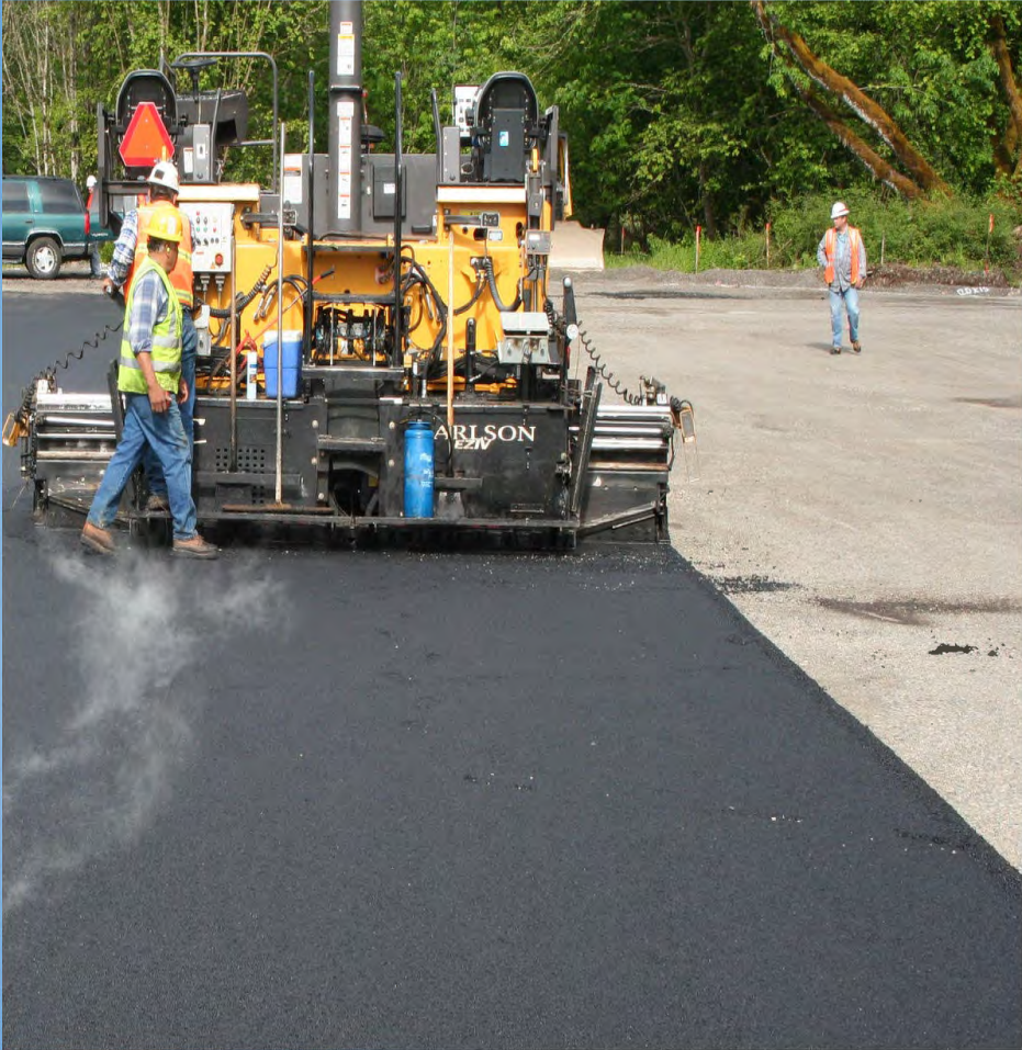
Admin/Excel Bldg Parking Lot
