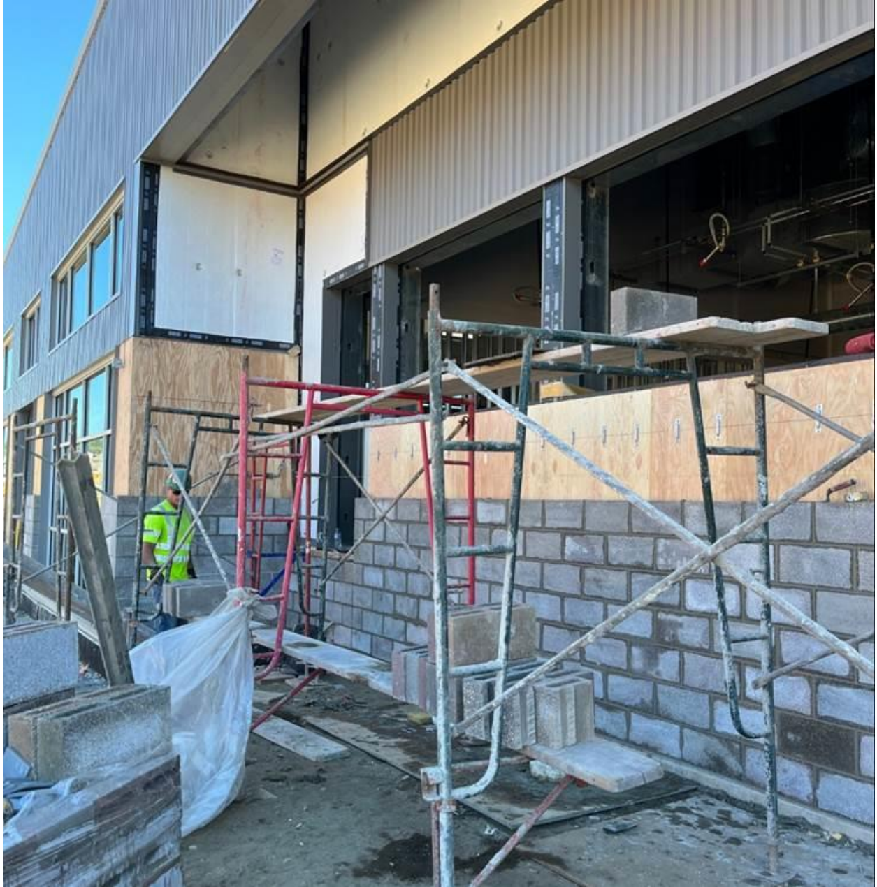
Masonry block around the CTE Wing is still being installed
