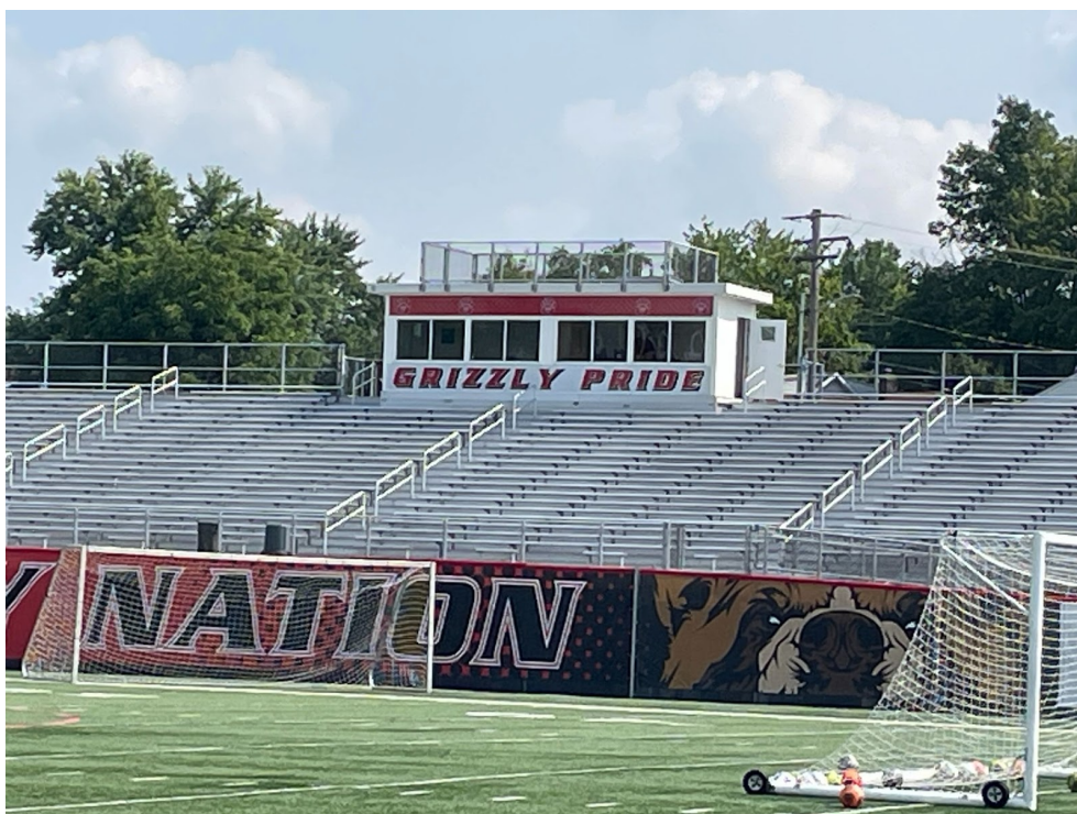
Front Side of the Visitor Press Box
