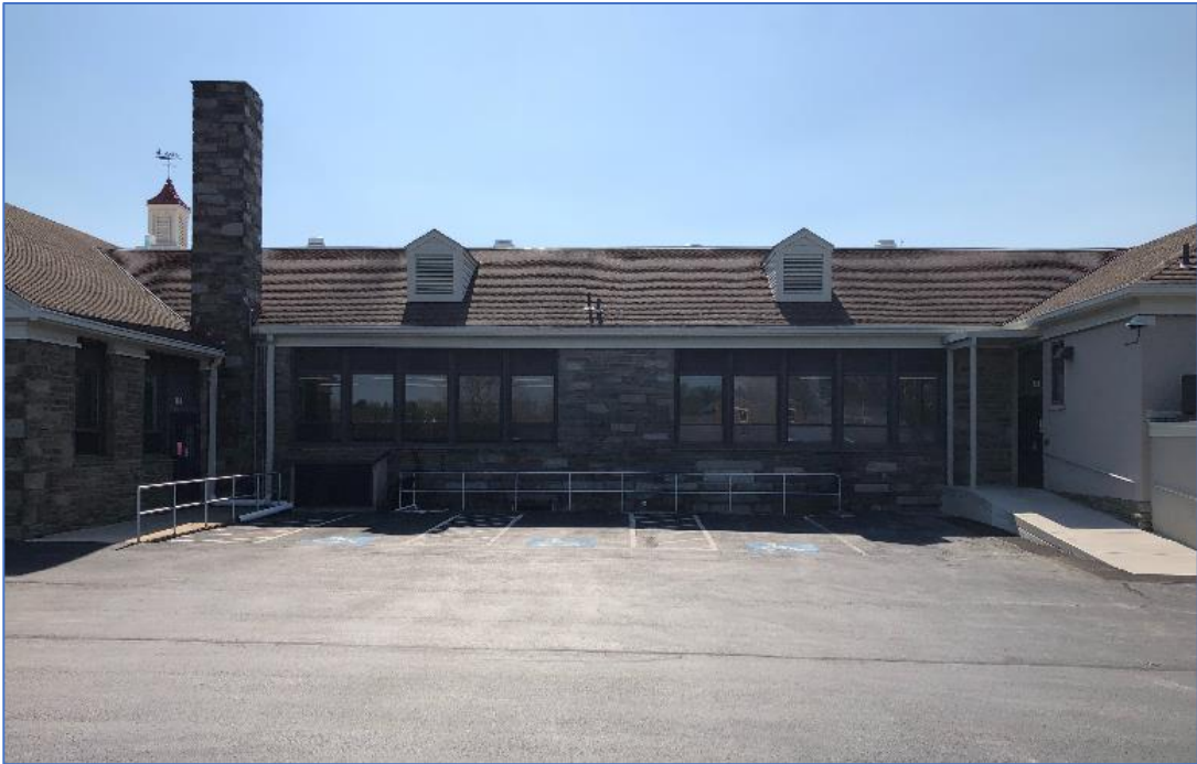
Photo #9: Great Valley School District Office, northeast (rear) elevation, 1939 building. 2021. Camera facing southwest.
