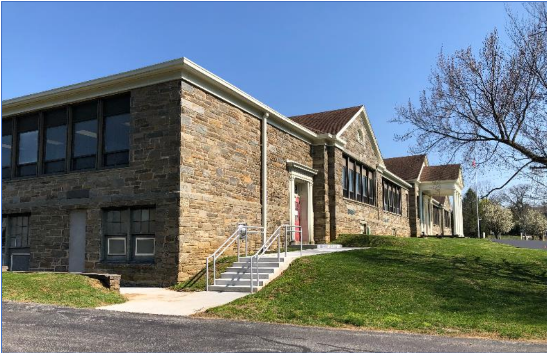
Photo #5: Great Valley School District Office, west corner, 1951 addition (left). 2021. Camera facing east.
