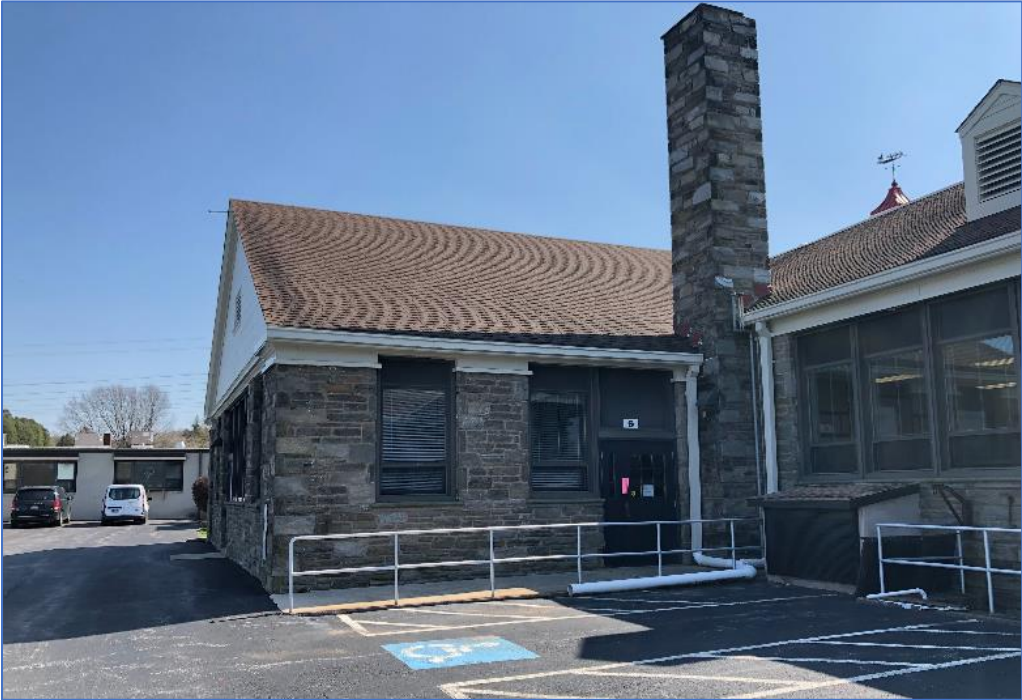
Photo #11: Great Valley School District Office, 1939 building (rear). 2021. Camera facing southeast.
