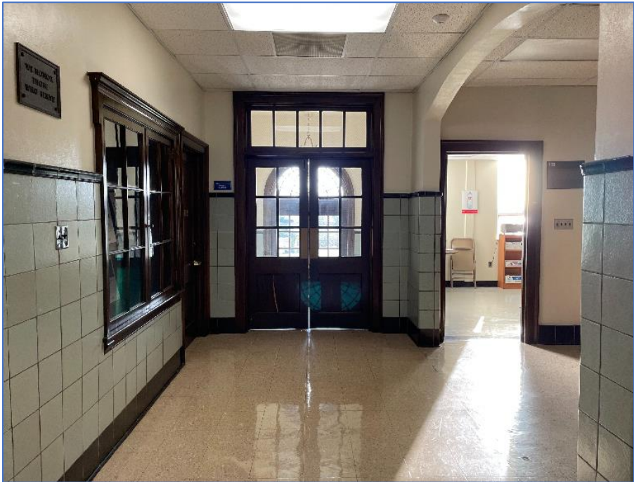
Photo #21: Great Valley School District Office, main entry foyer looking to vestibule. 2021. Camera facing southwest.
