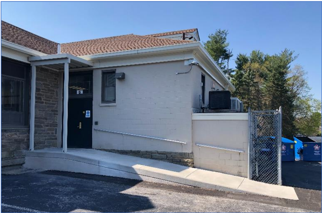
Photo #10: Great Valley School District Office, 1951 addition (rear). 2021. Camera facing west.
