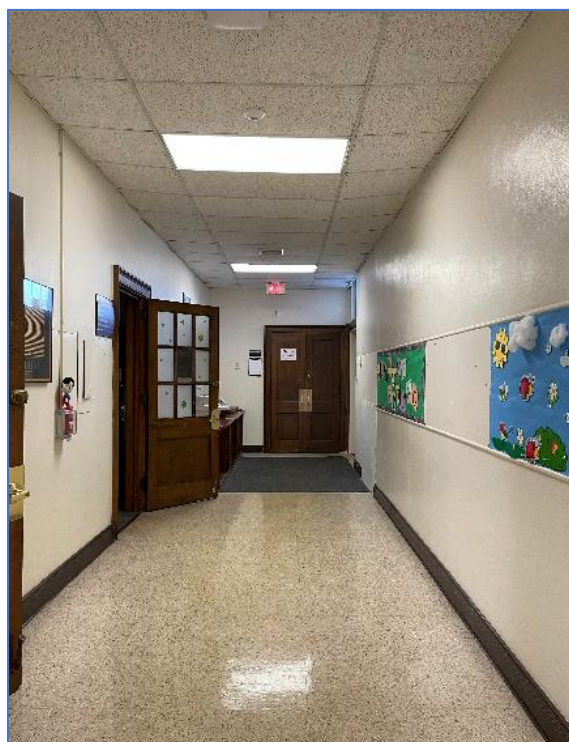
Photo #28: Great Valley School District Office, 1951 northwest addition corridor rear exit. 2021. Camera facing northeast.
