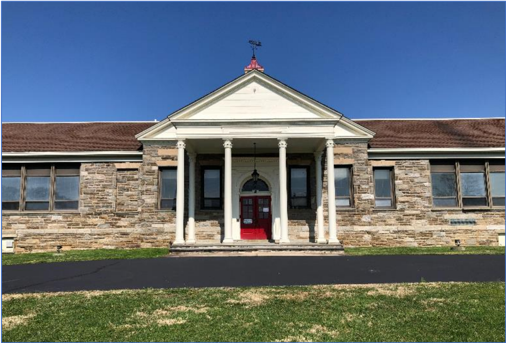
Photo #3: Great Valley School District Office, Southwest (main) façade, 1939 building, entryway. 2021. Camera facing northeast.
