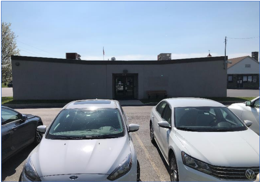
Photo #14: Great Valley School District Office, 1956 wing addition. 2021. Camera facing southwest.
