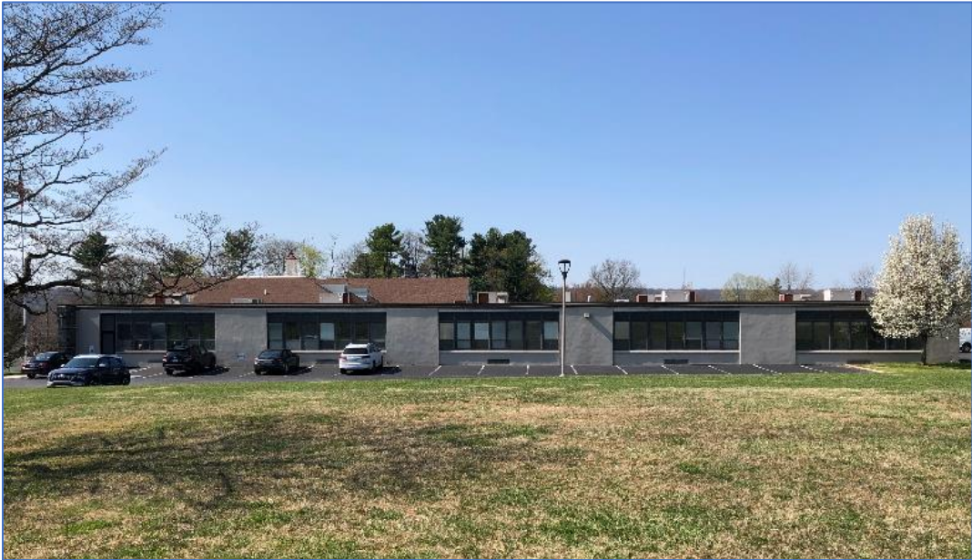
Photo #15: Great Valley School District Office, 1956 wing addition. 2021. Camera facing northwest.
