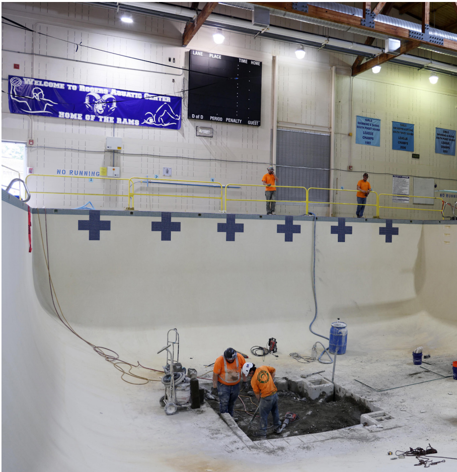
The crew members from Evergreen Concrete Cutting, Inc. remove the plaster and concrete from Rogers High School Pool to expose the filter system and drainpipes below the surface.
