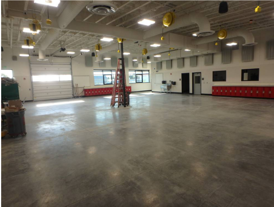
Looking southeast across the shop
