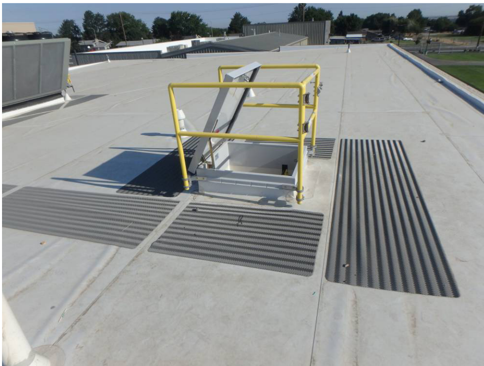
Roof hatch and railings
