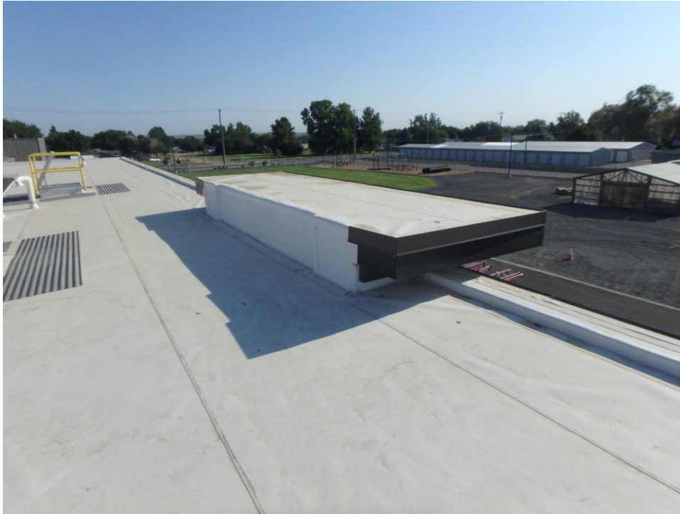
Main entry overhang
