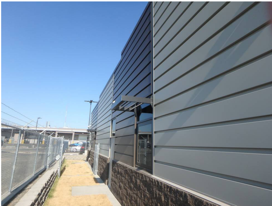
Looking west along the South elevation
