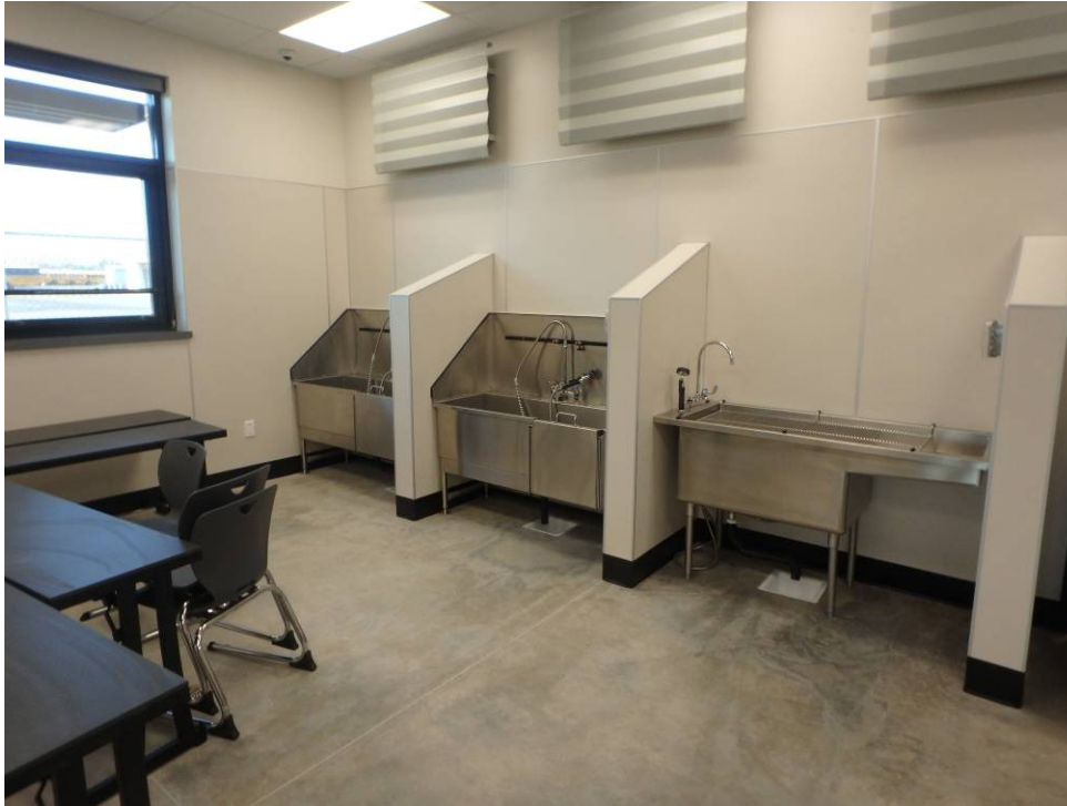
Lab dogwash stations and acoustical panels
