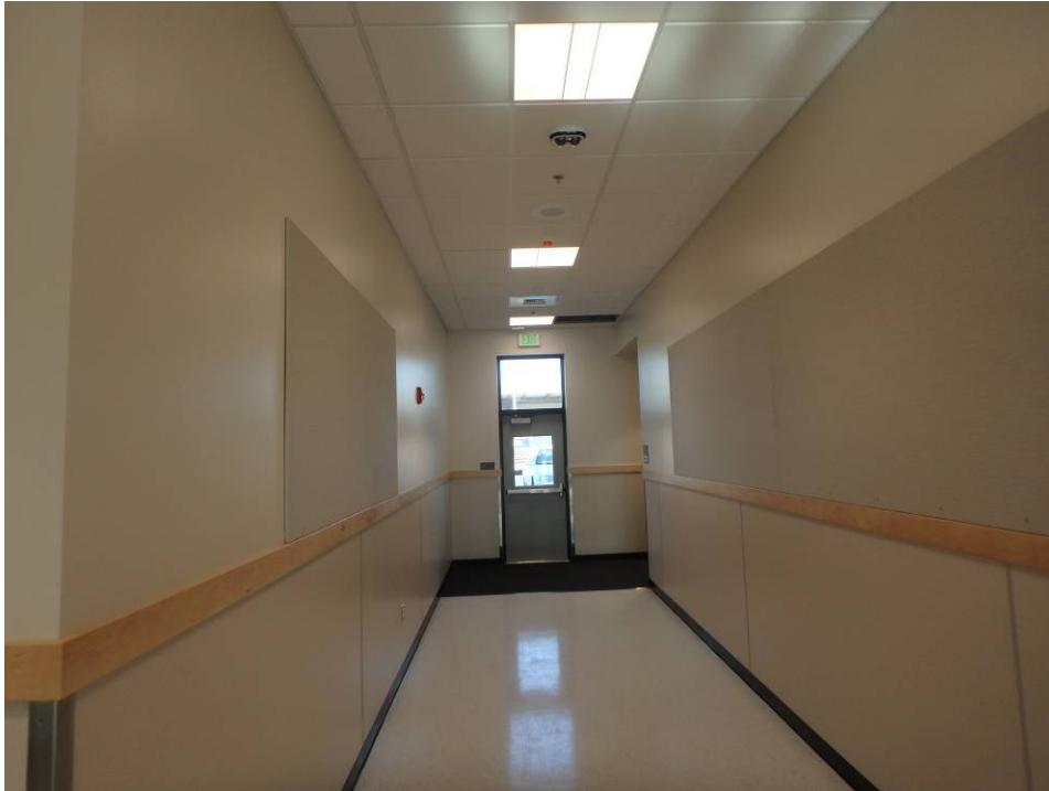
Looking west at the main east-west corridor
