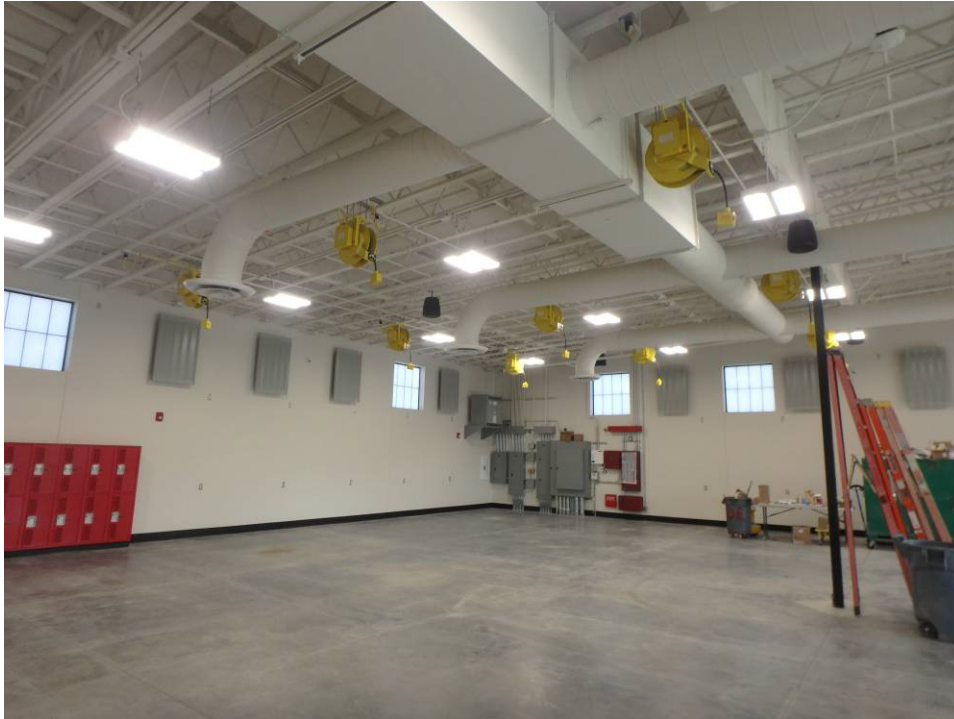
Looking NNW at the west half of the shop
