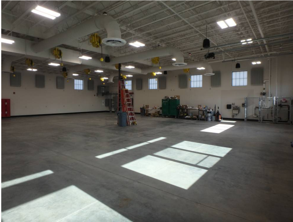
Looking northwest across the shop
