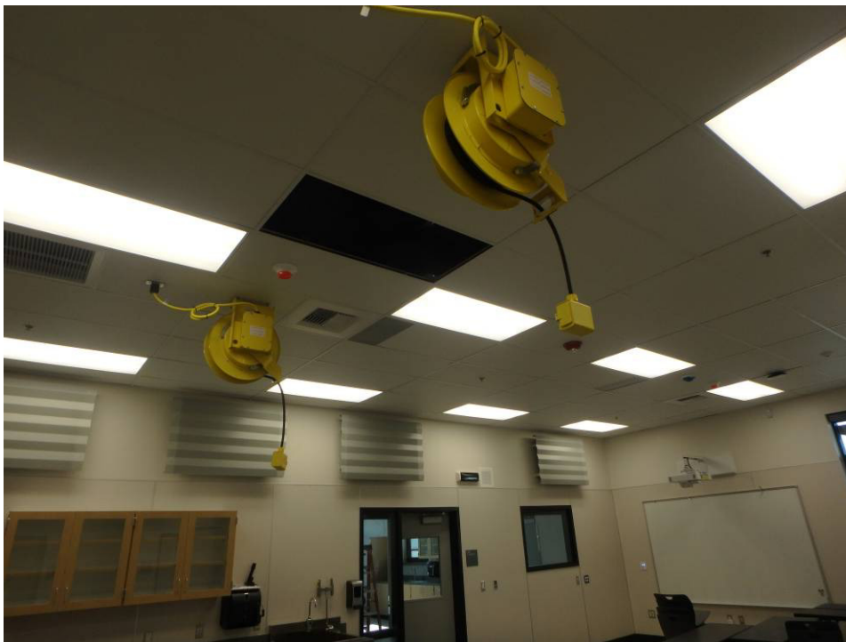
Lab cord reels and acoustical panels
