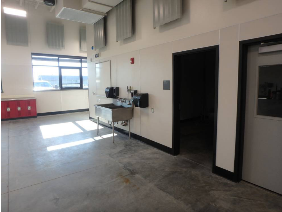
Shop's south sink
