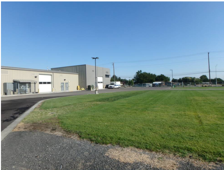
Looking north along the central curb
