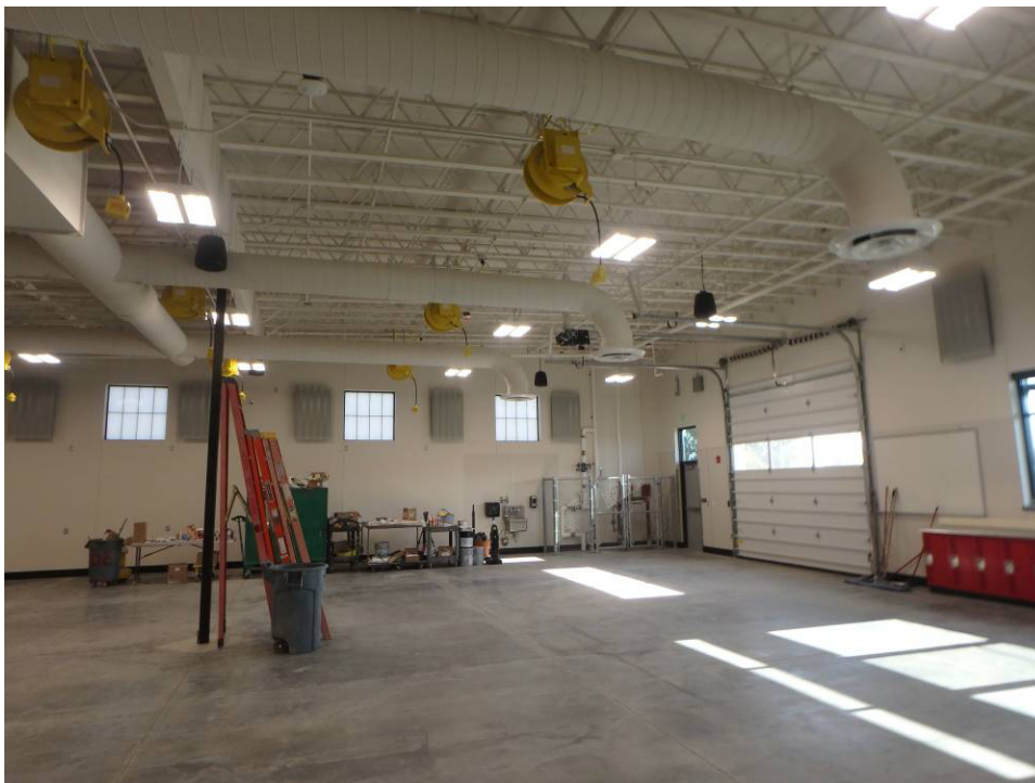
Looking NNE at the east half of the shop
