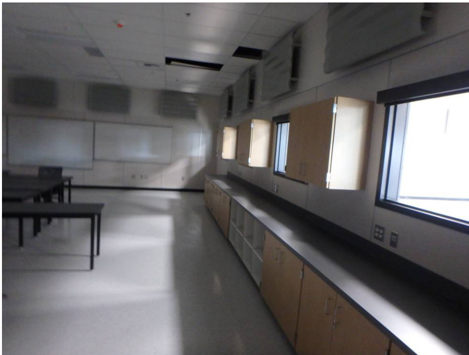
Looking west along the north classroom's north wall
