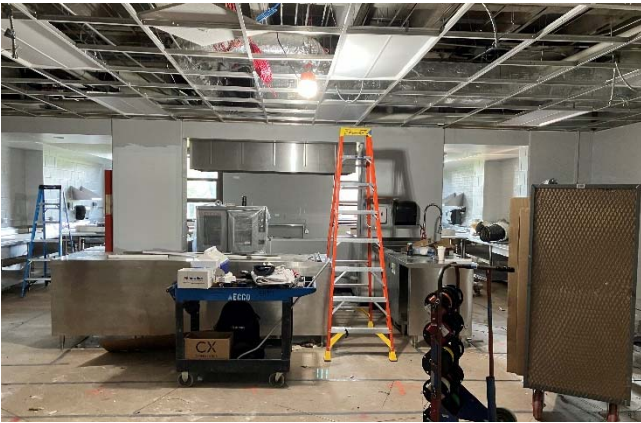
Left: FACS kitchen classroom 116 with new lights, ceiling grid, and paint.
