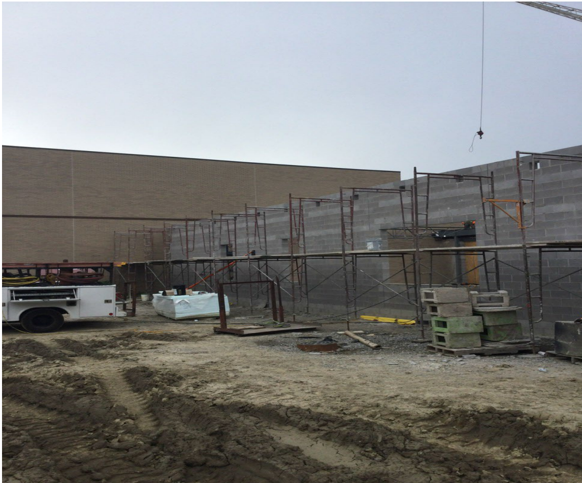
Block Going Up in Courtyard
