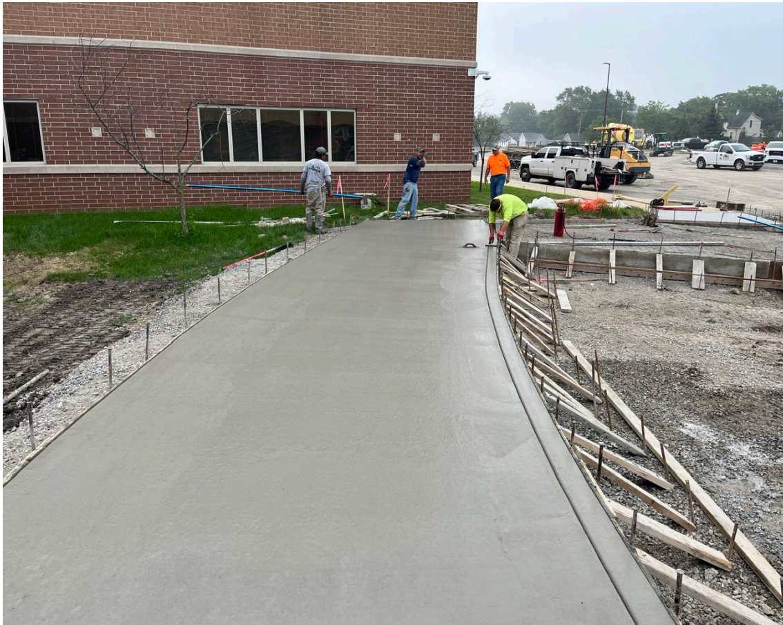
Sidewalk Poured Leading to New Auditorium
