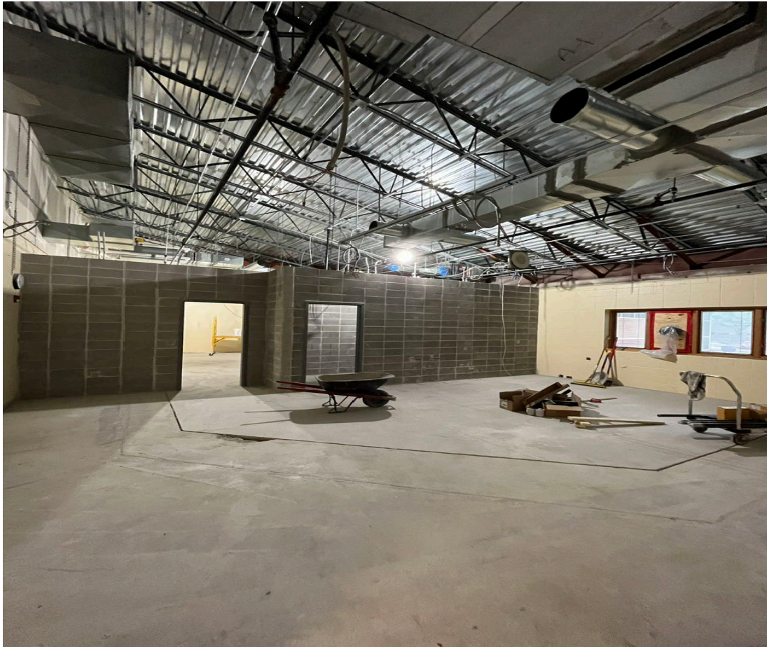
Installing Exterior Classrooms Walls
