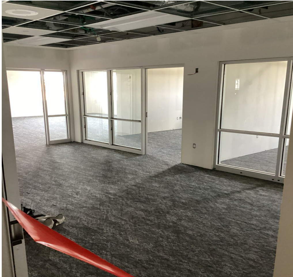
Inside Office View
