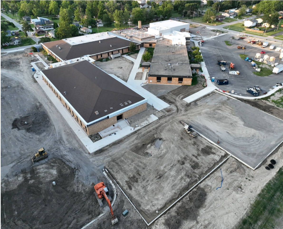
Aerial View of Entire Building
