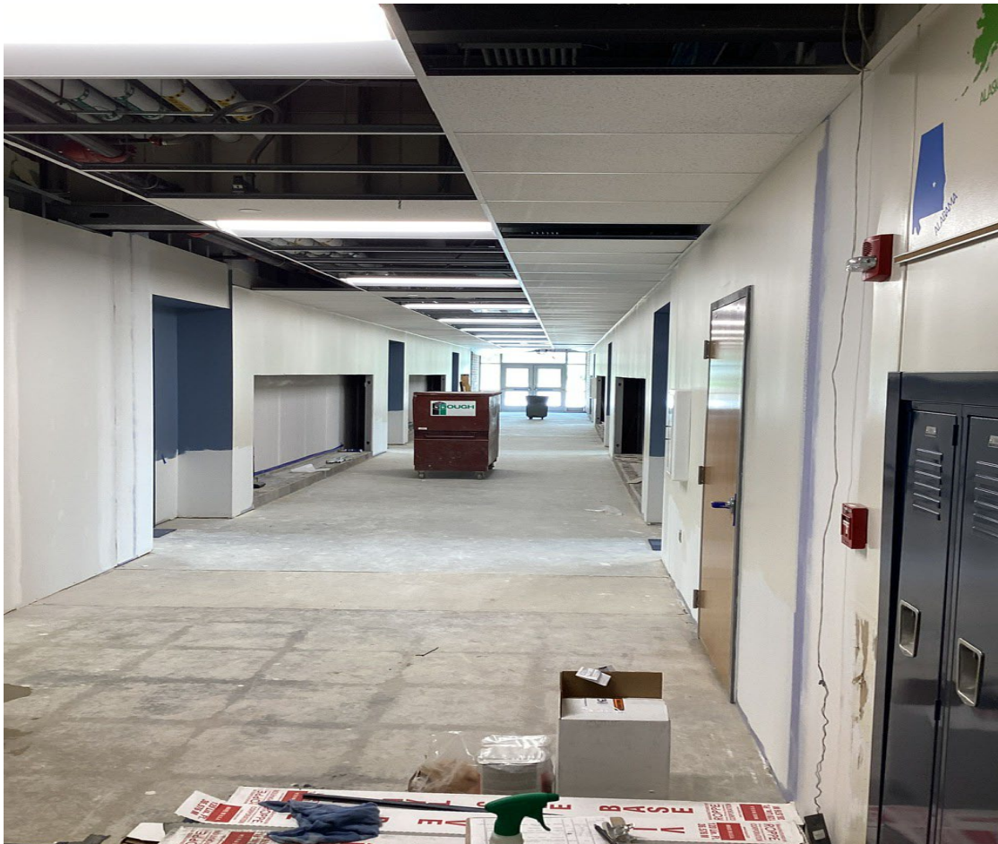
Unit E Corridor Renovation
