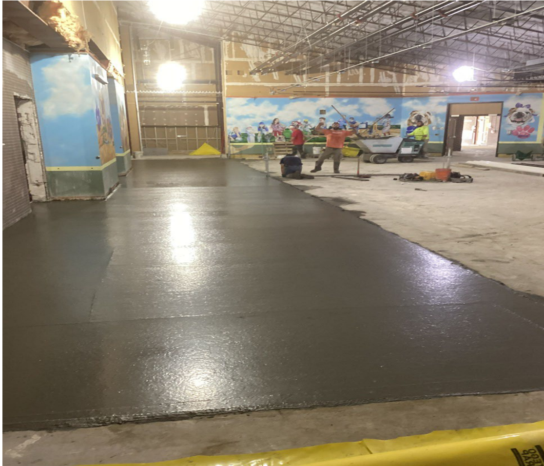
Completed Pouring Concrete in Kitchen
