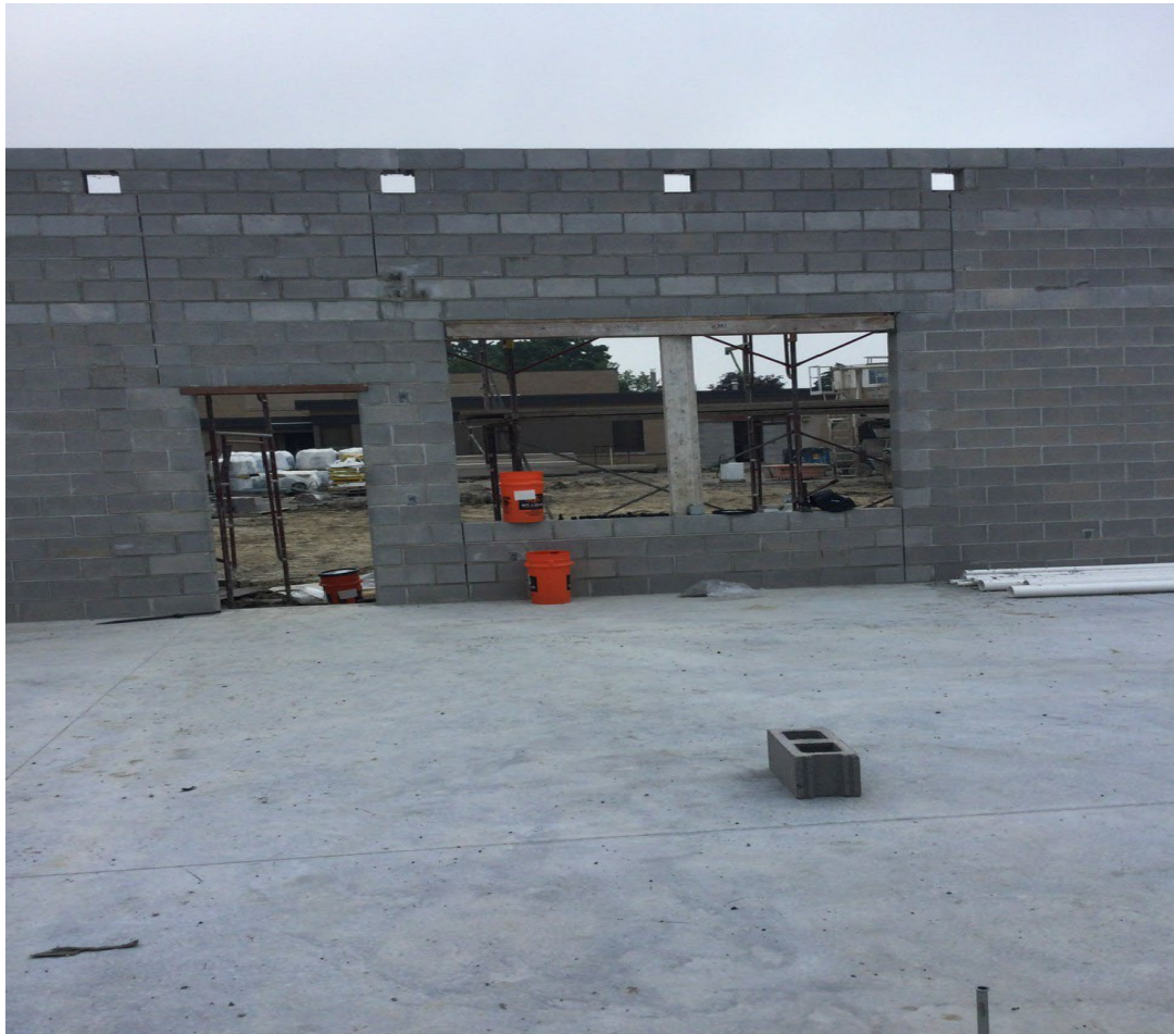
Additional Block Work in Courtyard
