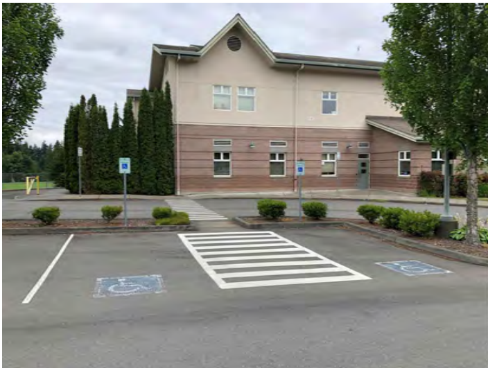
From ADA stall in south parking lot, continue over the crosswalk, and use the curb cut to gain access to the sidewalk. Follow this sidewalk north for building access.
