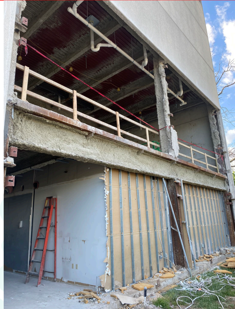
Exterior precast panels completely removed
