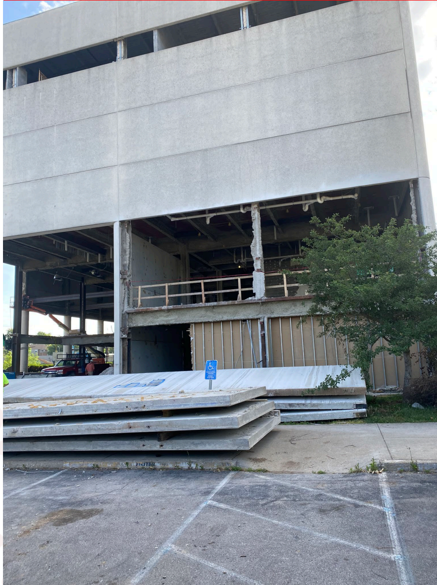
Exterior precast panels completely removed
