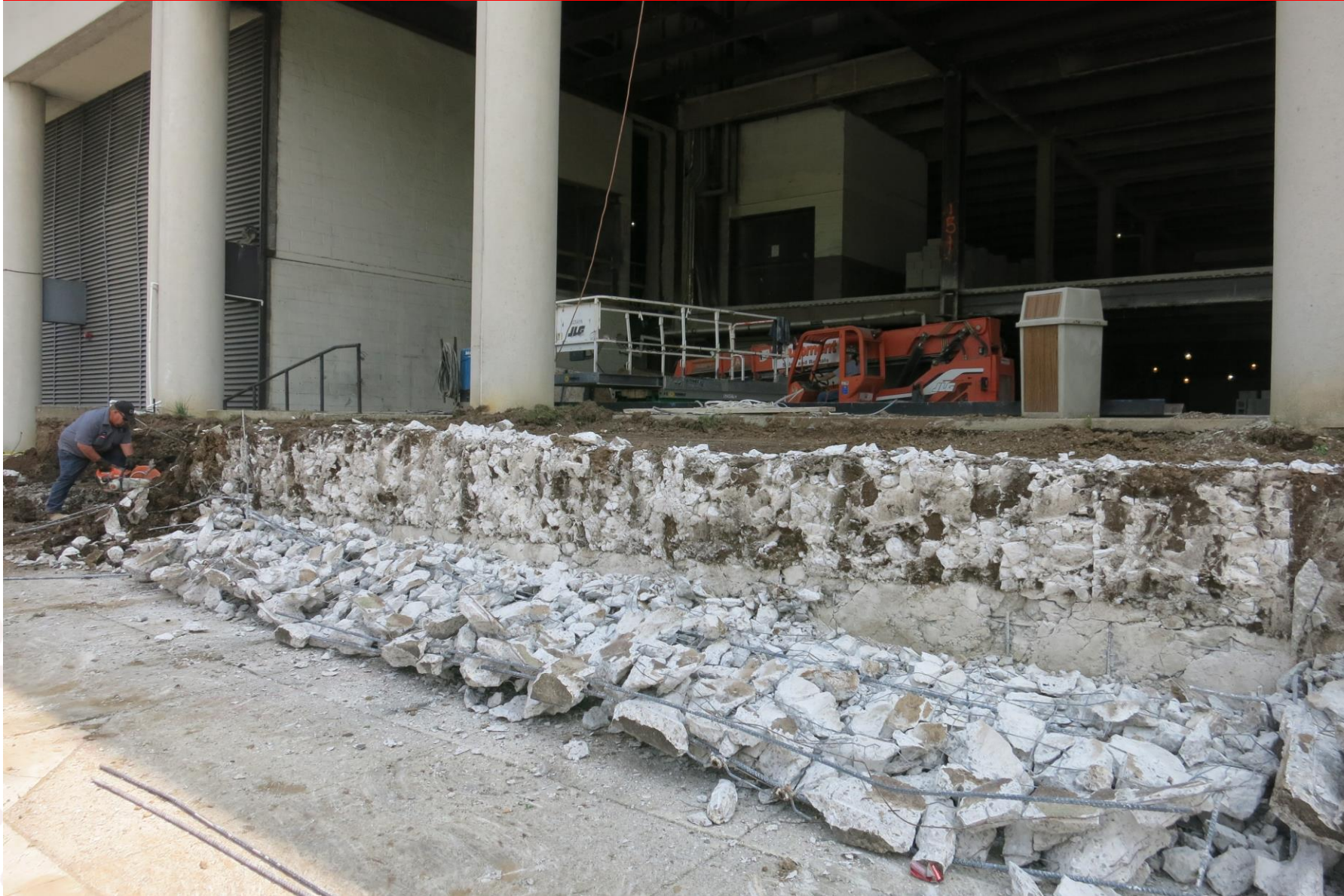
Portion of retaining wall planter being removed and shrubs
