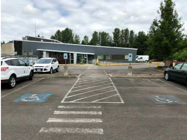
From ADA stalls continue on the hatched area to the nearest door for building access to EdTec.
