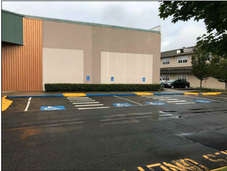
From ADA stalls, follow the curb cut to the main entrance for building access.
