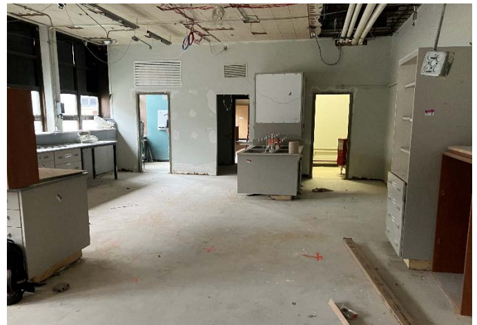
Right: Art classroom 218 stripped down. Art rooms 218, 212 and 210 will get durable epoxy flooring.
