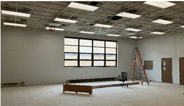
Left: Music room 169 getting ready for new ceiling and flooring.
