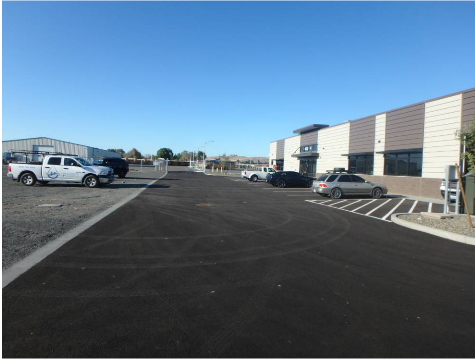
Looking south along the central curb
