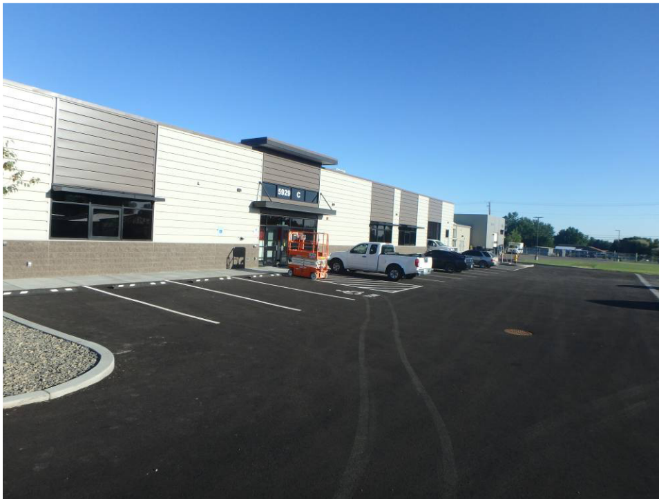
Looking north at the East Elevation
