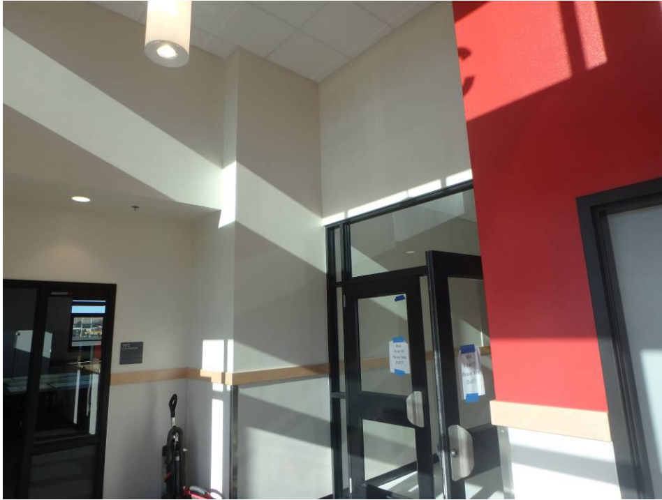
Inner vestibule doors to the east-west corridor
