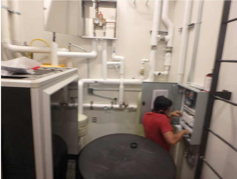
Mechanical room –north wall
