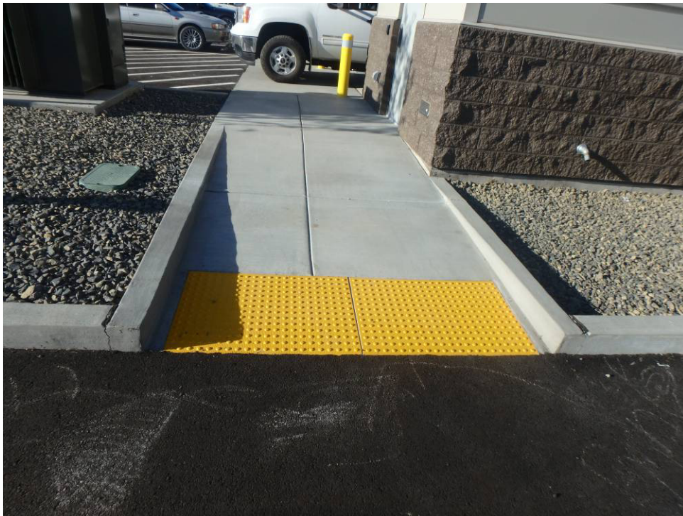
North sidewalk ramp
