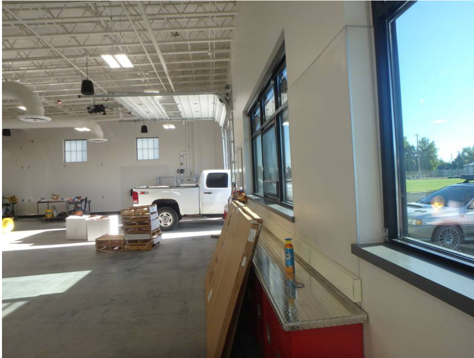
Looking north along the shop's east wall and lockers with diamond plate top
