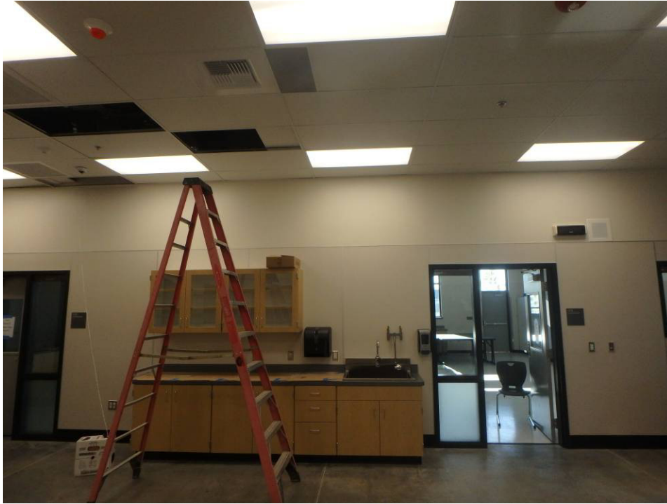
Lab – eyewash station and east wall
