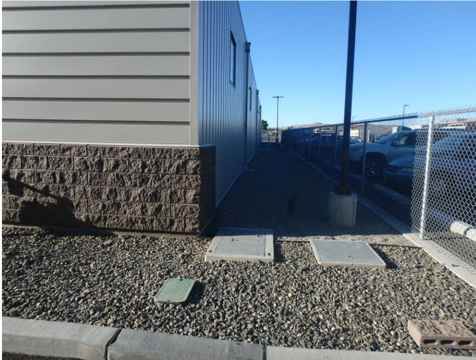
Looking south along the west edge of the building
