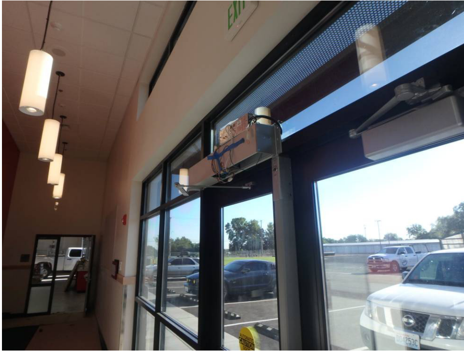
Looking north at the main entry doors
