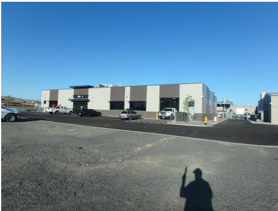
Looking southwest at the East Elevation
