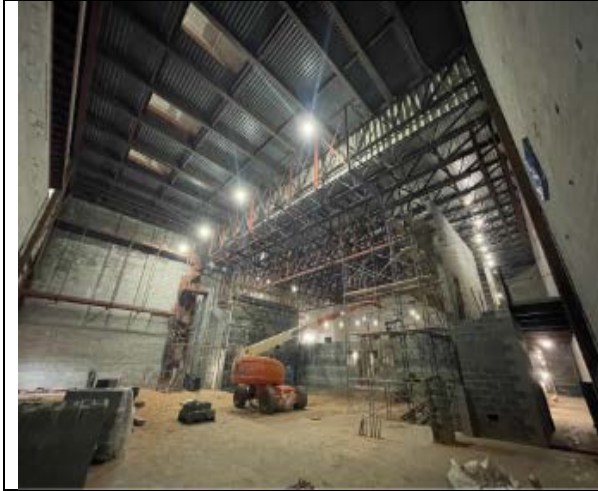
Auditorium Catwalk Steel
