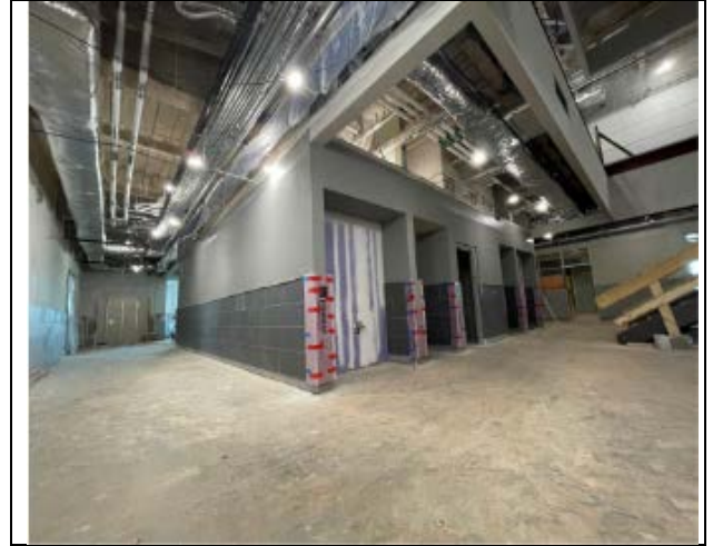
Area A Paint & Tile
