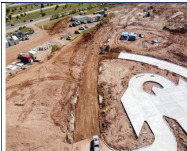
Entry Loop Subgrade and Paving
