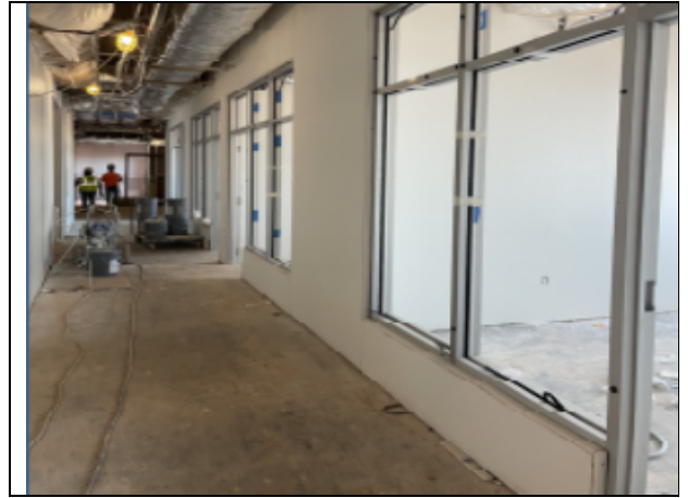
Interior Storefront Installation
