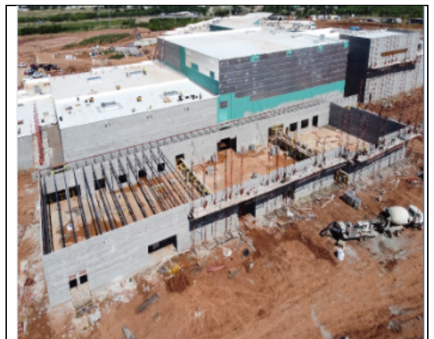
Steel and Masonry Areas J & M
