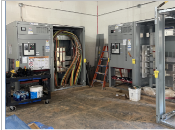
Main Electrical Room Buildout
