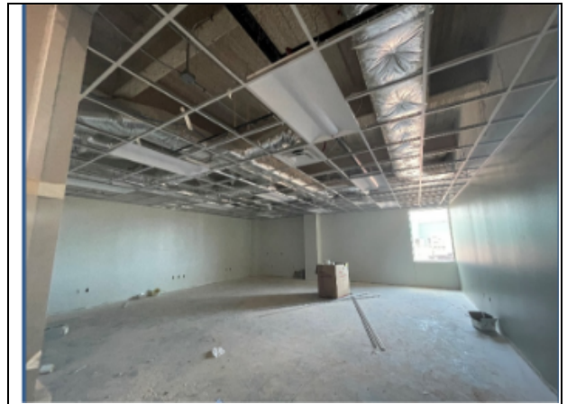
Area D Light Fixtures and Grid Ceiling
