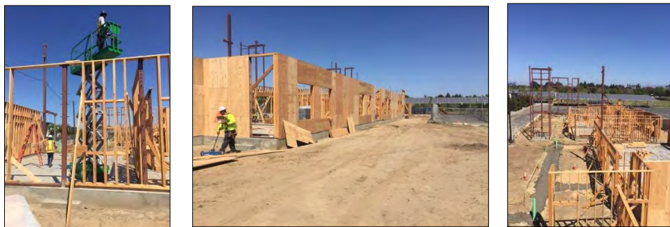
Marshall New Classroom Building Construction Progress – May 2018
