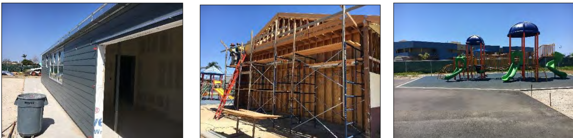
Harrington Child Development Center/Kindergarten Annex Construction Progress – May 2018
