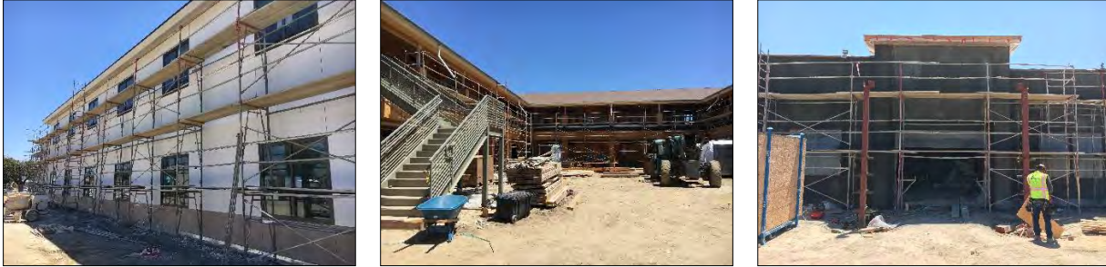
New Elm School Construction Progress – May 2018
