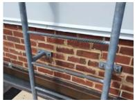
**EB-3 Brick Repairs**Brick veneer has pulled away at ladder. Brick veneer needs to be removed and rebuilt.
