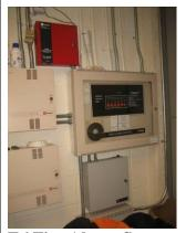
E6 Fire Alarm System: Replace fire alarm system with new due to end of life. The capacity has reached its limit.
