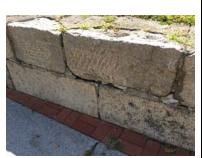
SS 1 Stone Site Wall: Restore and rebuild stone site walls. Reset loose stones and remove and replace deteriorated mortar joints.
