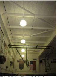
E1 Main Gym Lighting: Replace existing gym lighting with new. Broken and cracked lamp sockets were found.
