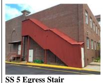
The corrugated metal walls of the exterior egress Stair enclosure are rusting and damaged. Replace existing metal stairs and walls with new stairs and enclosure that would be opaque partially to allow for natural light during the day.
