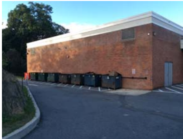
SS 15 Relocate Dumpsters Dumpsters adjacent the building create a potential health and fire hazard. Work would include relocating the dumpster area to away from the building on a concrete pad enclosed by chain link fencing for protection from vandalism
