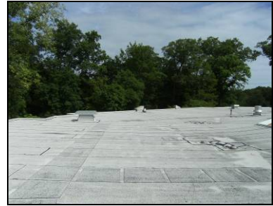
M13 Classroom Air Relief System (2003 Addition) Provide ducted powered exhaust to replace the existing rooftop plenum vent system.
