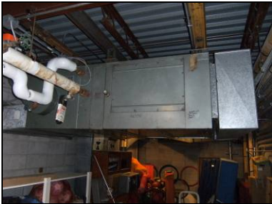
M8 Gymnasium air handlers Replace existing units.
